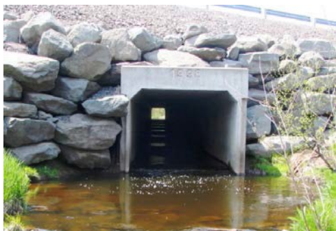
Figure 8. Example of a concrete box culvert.
