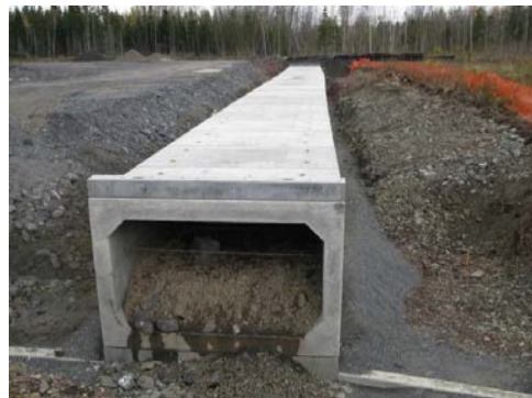
Figure 5. Example of an embedded culvert.
