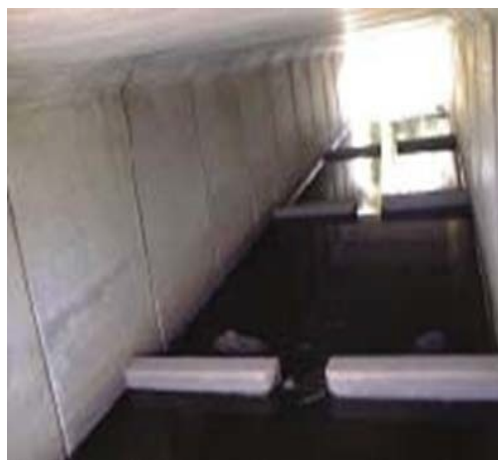
Figure 19. Example of baffle spacing
