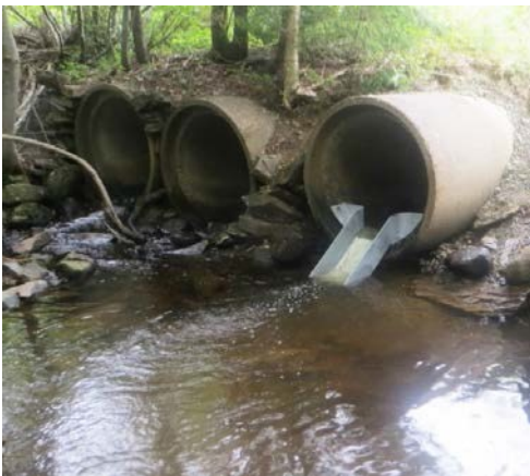
Figure 25. A chute installation on a culvert
