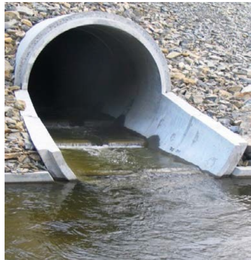
Figure 7. Example of a circular concrete culvert with baffles.
