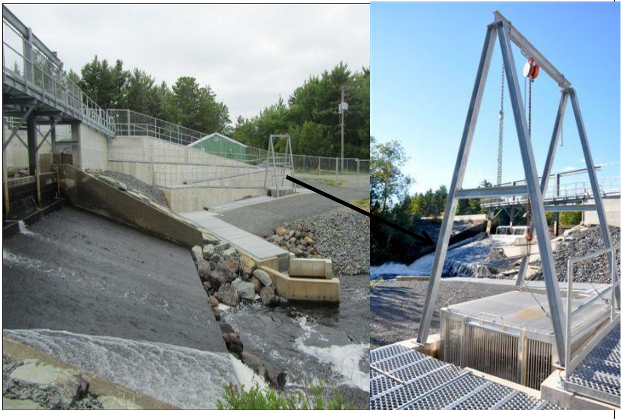
Figure 4. Hebb Dam fish passage facility. Left photo shows side view of dam and position of fish trap in one of the lower pools. Right photo shows close-up of fish trap partially raised.
