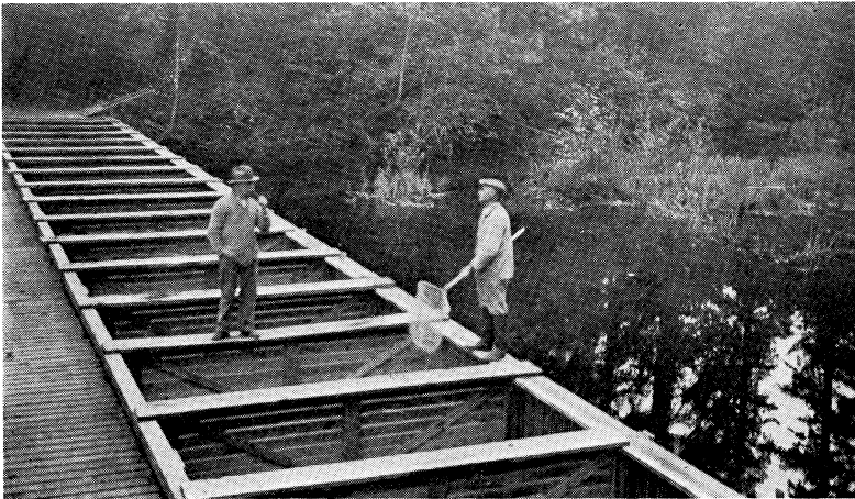
FIGURE 3. An end view of the adult salmon counting fence from above, showing the series of traps from which the fish are dipped for counting or stripping. The down-stream walls of the traps are constructed of pickets similar to the up-stream face. The whole structure, approximately 5 ft. high, rests on a solid, plank platform.
