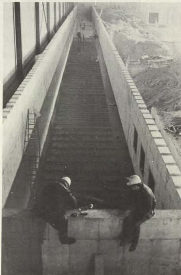
Figure 1. Towing tank under construction, February 1972
