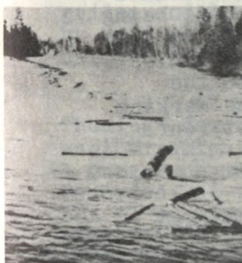
Fig. 5. Pulpwood and logs diverted by finboom to pass partial N.W. Miramichi fence during early part of smolt run, 1953.
