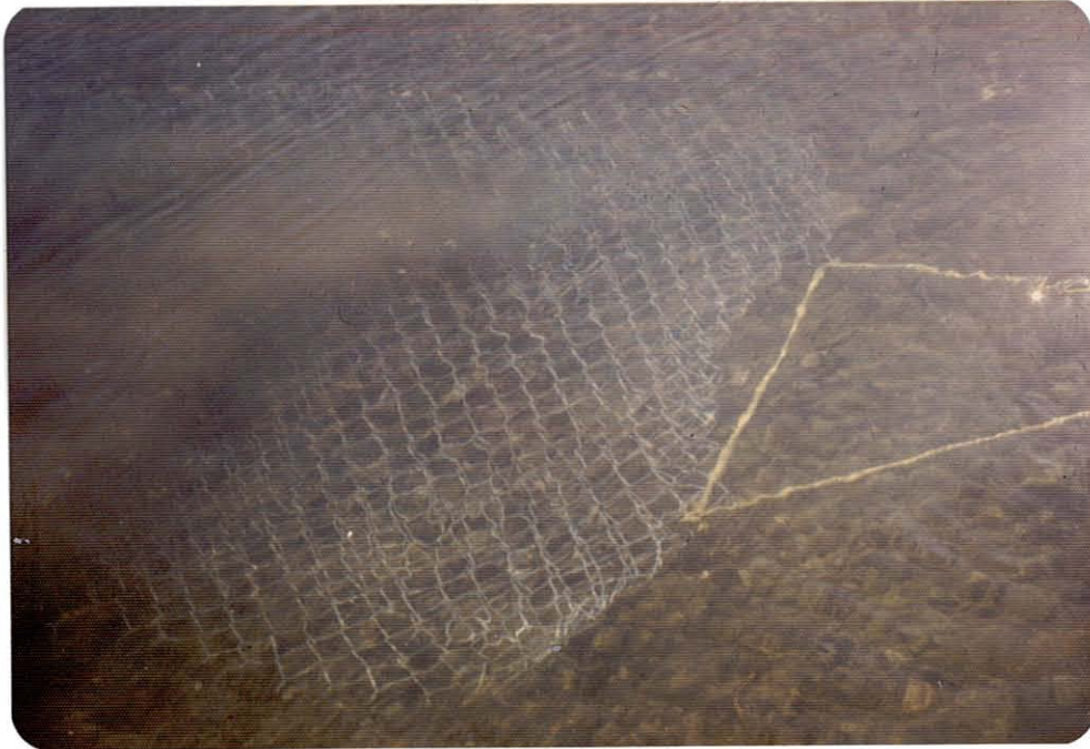
PLATES 7 - 8 PUNTLIDGE CHANNEL CLEANING MARCH 21, 1979
