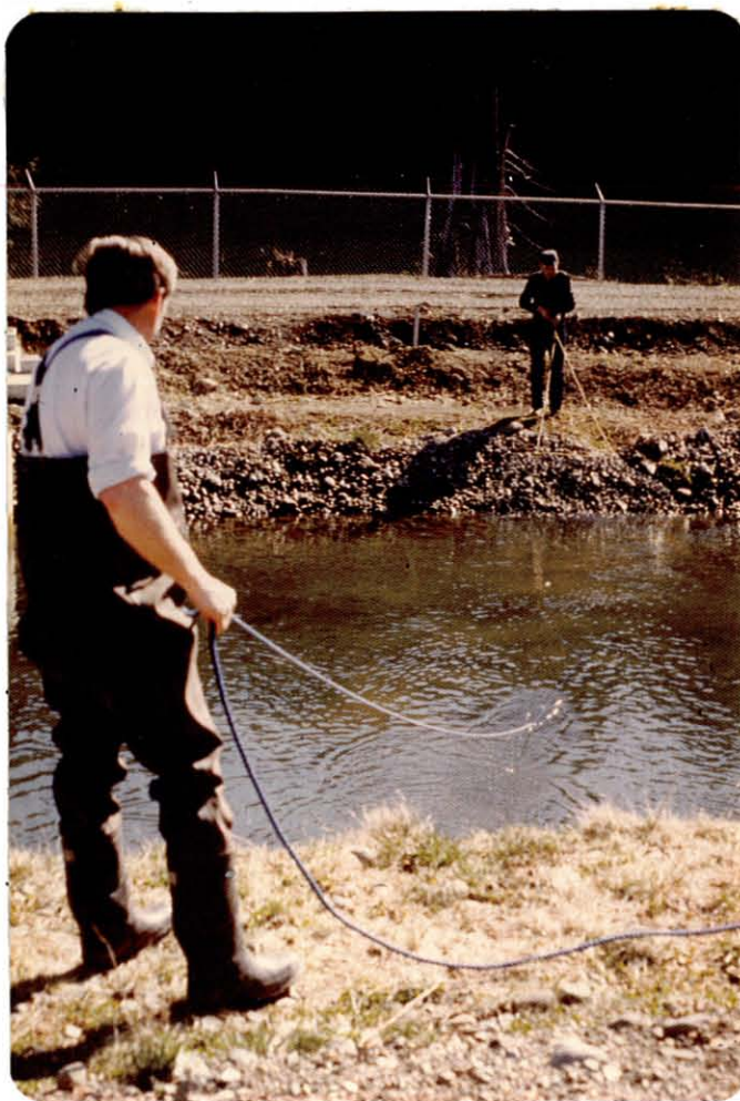
Plate 6. Cleaning procedure at Puntledge channel. Note section of chain link fencing is dragged across channel. March 21, 1979.
