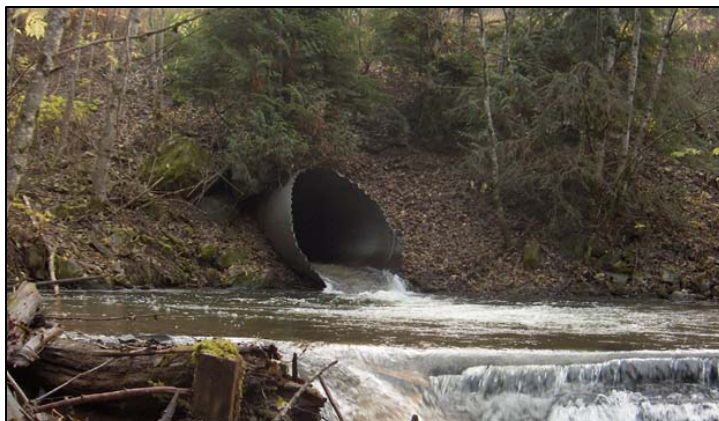
Figure 62. Singlehurst Creek culvert outlet.
