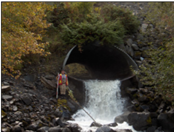
Figure 74. Highway 16-Shandilla Creek culvert. Outfall drop bars fish passage.
