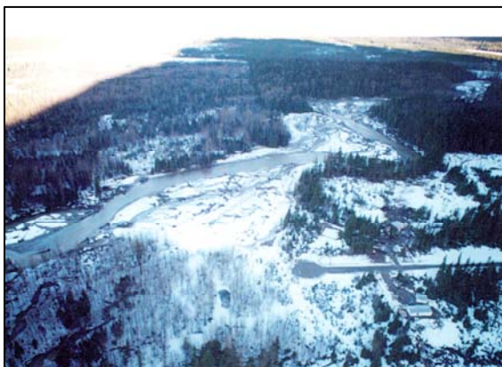
Figure 42. View of Williams Creek, reach 3, upstream portion.
