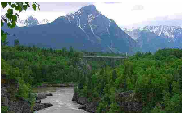
Figure 123. Hagwilget Canyon upstream of the bridge.
