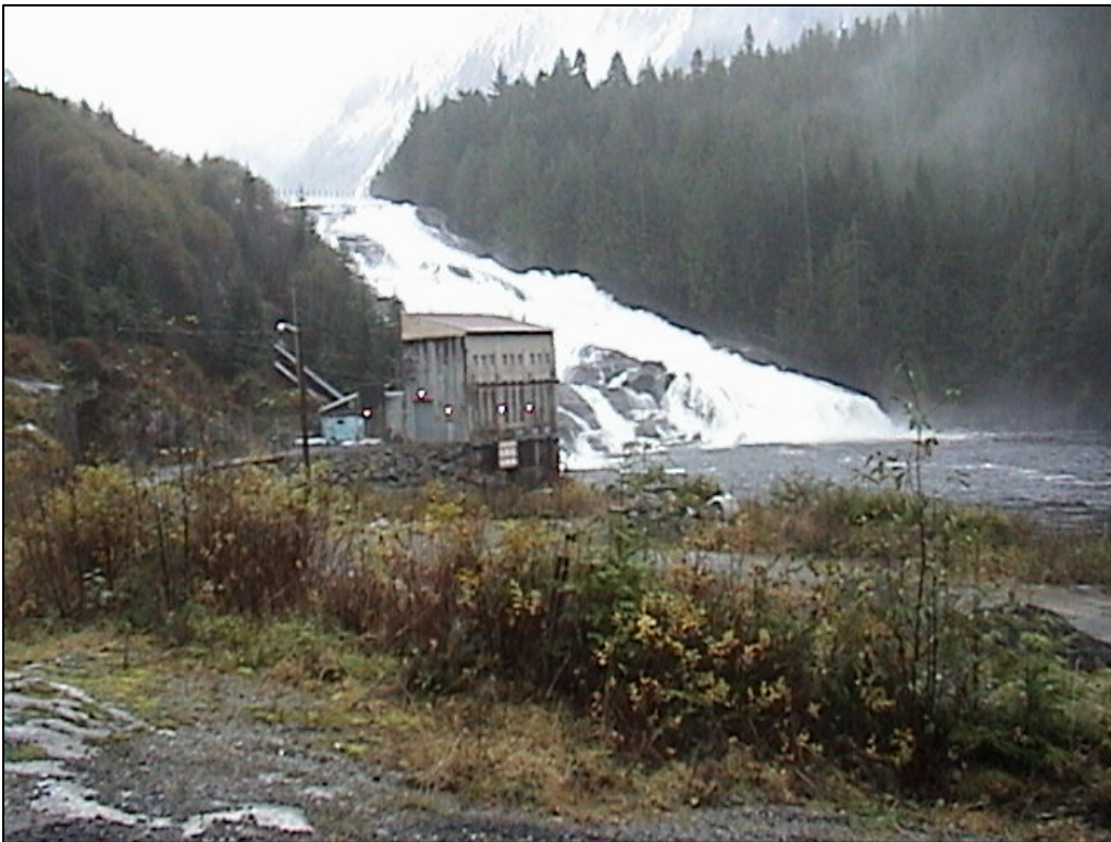
Figure 36. Big Falls River dam outlet.
