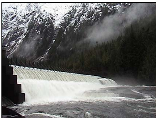
Figure 38. Falls River dam spillway. L. Miller.
