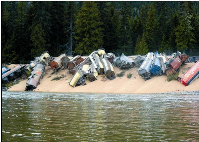
Figure 63. CN Rail grain units derailed into Skeena River, 2004.
