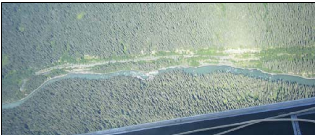
Figure 120. Large earth slumps into the Skeena River. These failures originate with the abandoned BC Rail grade. J.Allen
