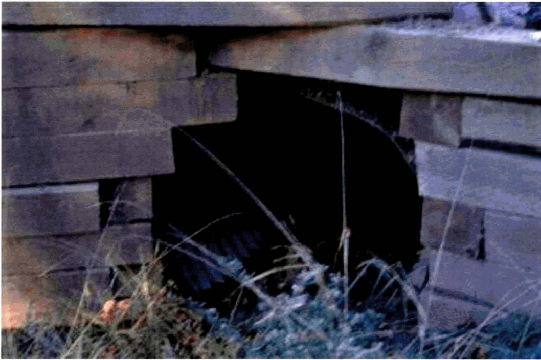
Figure 17: Innovative ideas for stabilization in difficult soils.
