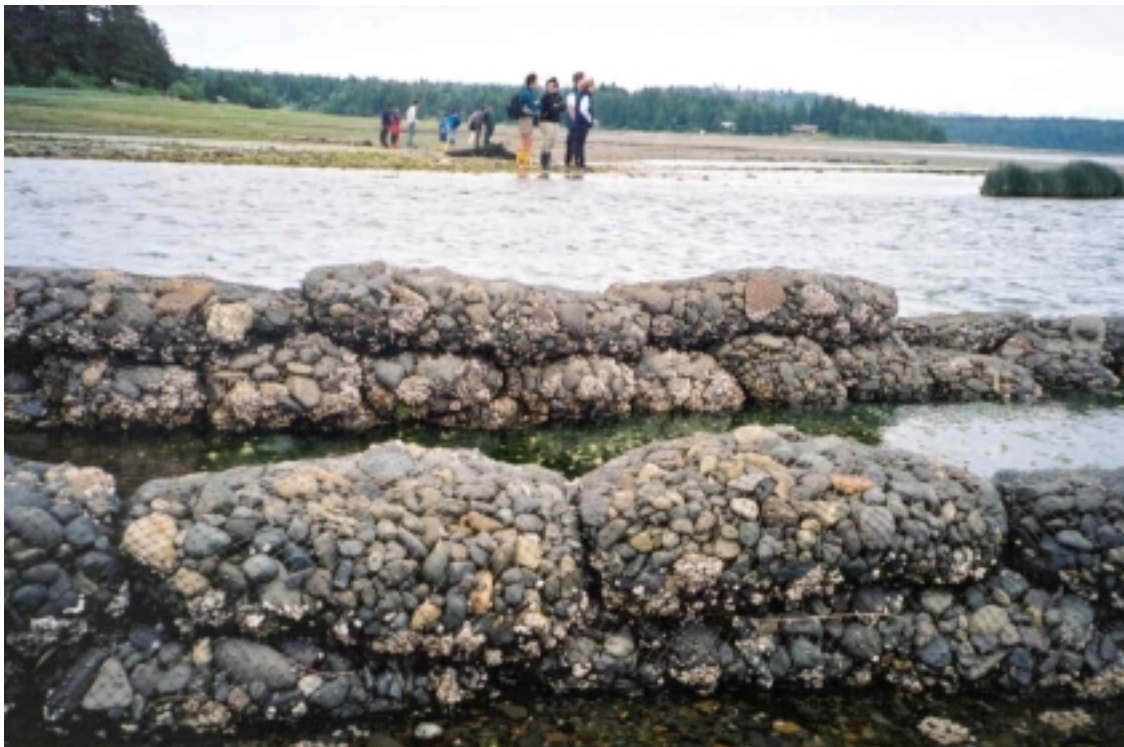
Figure 32: Gabions used for estuary channelisation at Wilfred (Coal) Creek
