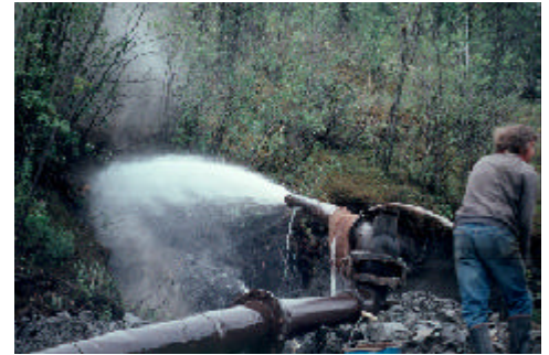
Washing the land to remove the "overburden"
