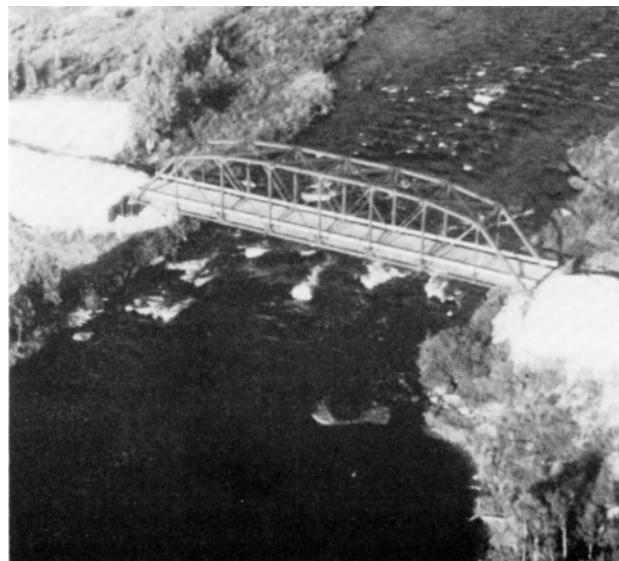
Fig. 5.1 Bridge on the Clearwater River
