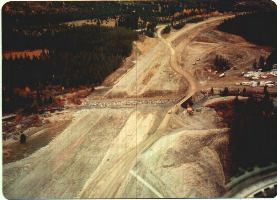
PHOTO 20. Coquihalla Highway bridge crossing showing river diversion and placement of rip rap along channelized stream section (Photo by G. Kosakoski).
