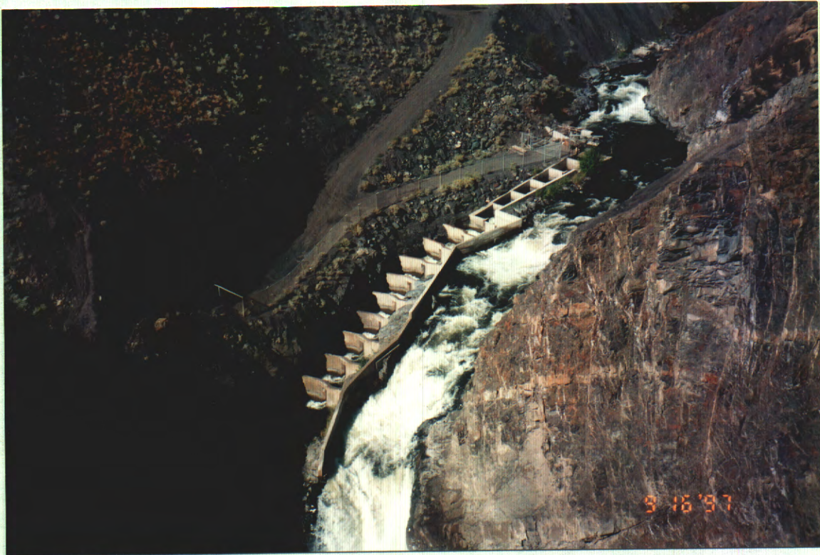
PHOTO 11. Overhead view of the Bonaparte River fishway constructed in 1989 (Photo by M. Crowe).
