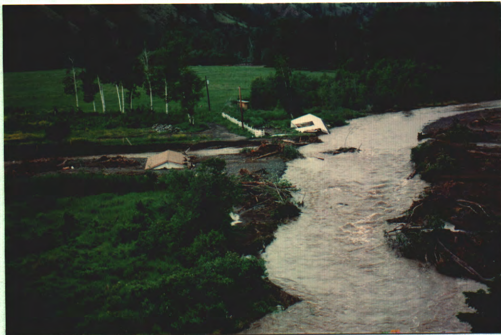
PHOTO 10. The June 1990 flood in the Deadman River destroyed the Deadman River hatchery (Photo by J. Patterson).
