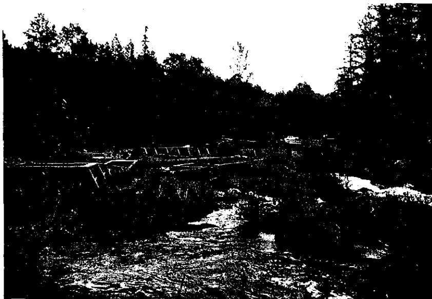
Downstream view of fishway at Skutz Falls.
