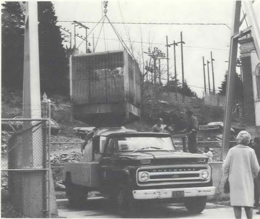
A pivoting steel basket is used to transfer salmon from a holding pool to a tank truck for transportation to breeding grounds in the upper part of East River.
