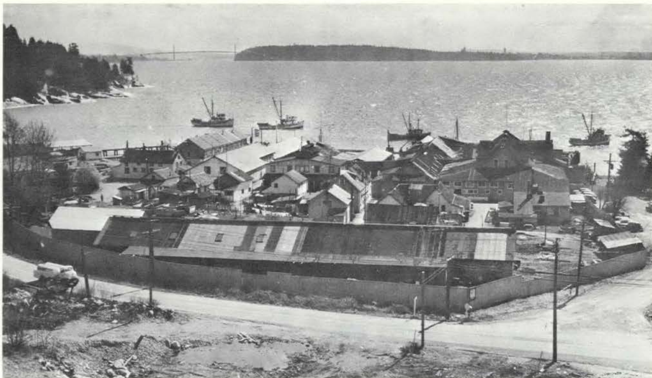
This is the Francis Millerd and Co. Ltd. cannery on Marine Drive, West Vancouver, recently purchased by the federal Government as a site for a Fisheries Research Board of Canada's water laboratory. The site will be developed as a research centre over the next 10 years.
