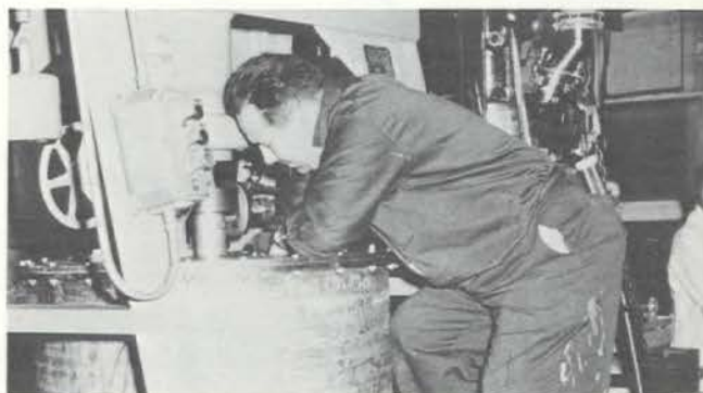
Basket centrifuge is used to separate fish from alcohol-water-fat mixture.
