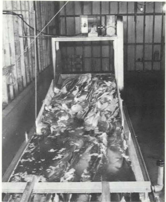
Thawed flounder being conveyed up the discharge ramp of the water thawer located at the Catalina plant of Fishery Products Limited.
