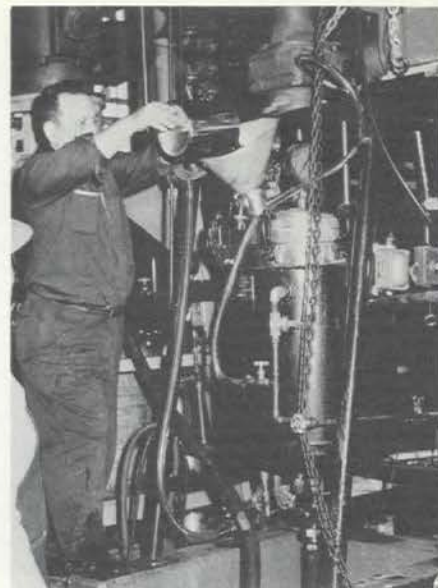
The fish-alcohol mixture is put in steam heated extraction kettle.
