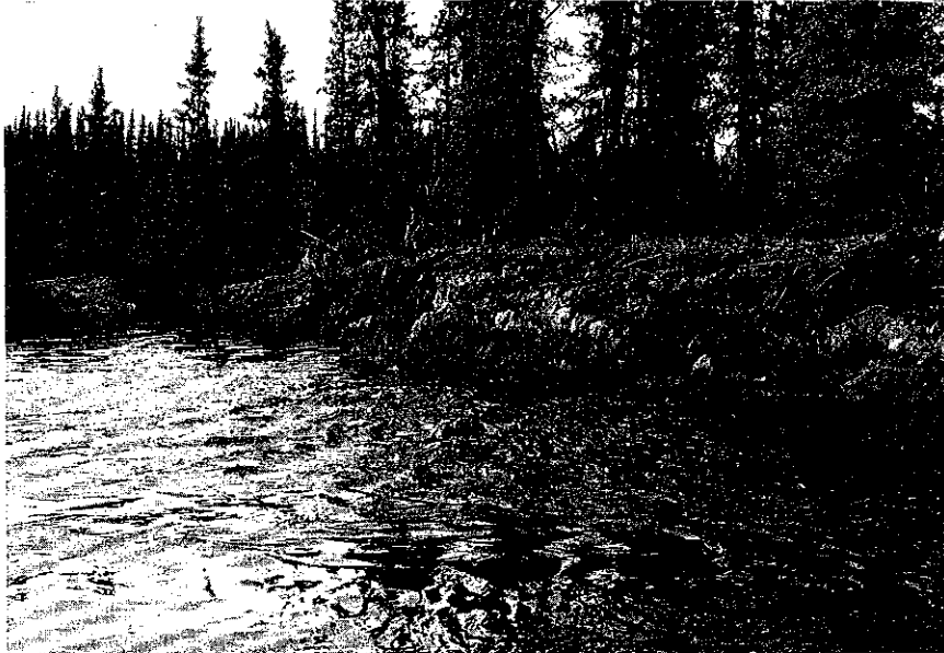
Block slumping occurring along left bank of the Sekulmun River approximately 400 feet upstream of hub P30.
