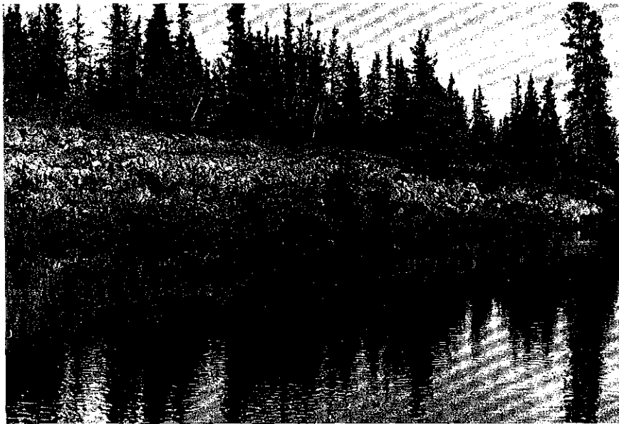
Sloughing of left bank of the Sekulmun River near hub P40.
