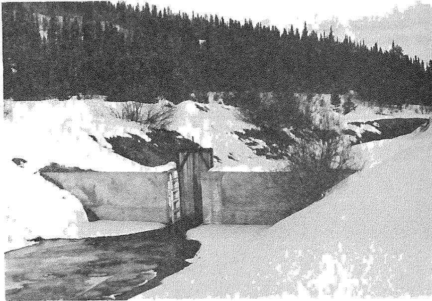
Plate 81. Jackson Lake control structure (north).
