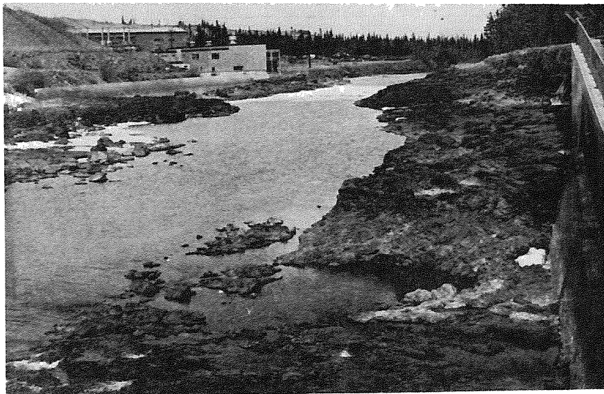
Plate 88. Downstream view of the transportation channel at low water levels (1973).
