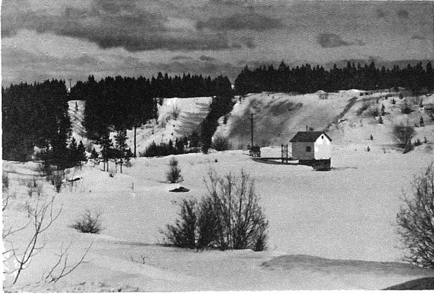
Plate 78. McIntyre Creek control structure.
