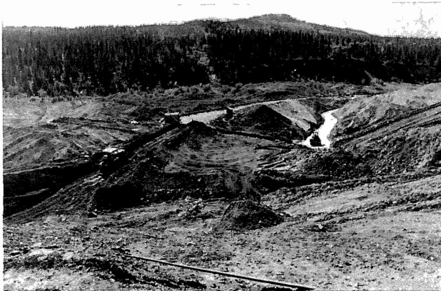
Plate 8. Pine Creek- hydraulic mining (gold).
