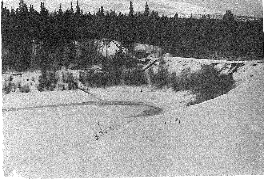
Plate 80. Jackson Lake control structure (south).
