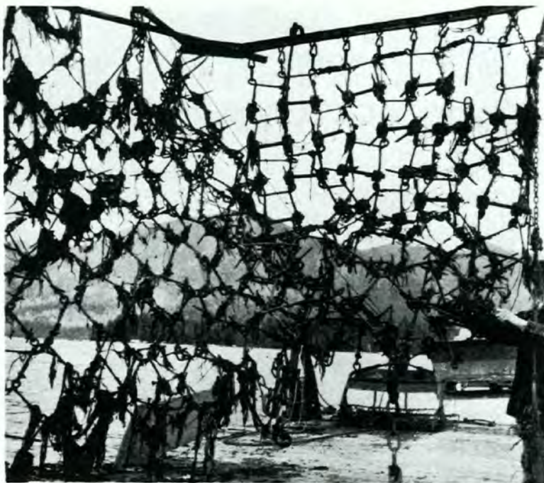
FIG. 80. Spring-toothed harrow used for breaking clusters of oysters.
