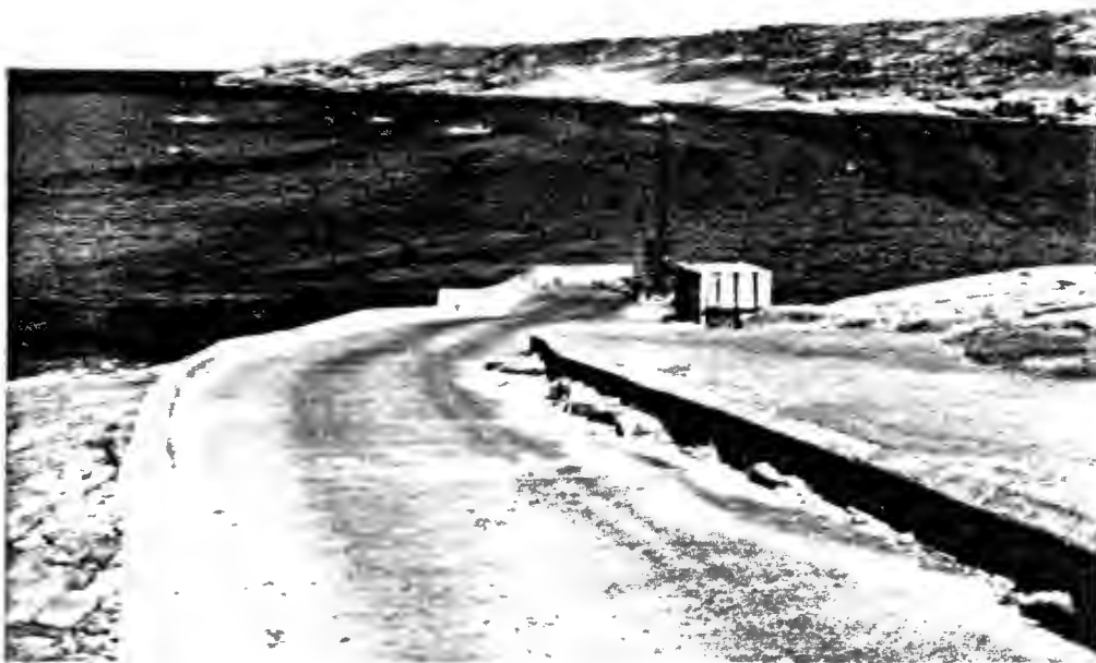
2. Martin's Point Landing Wharf and Approach
