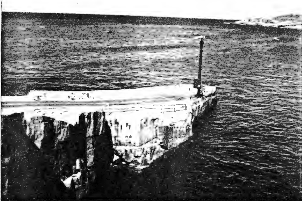
1. Martin's Point Landing Wharf
