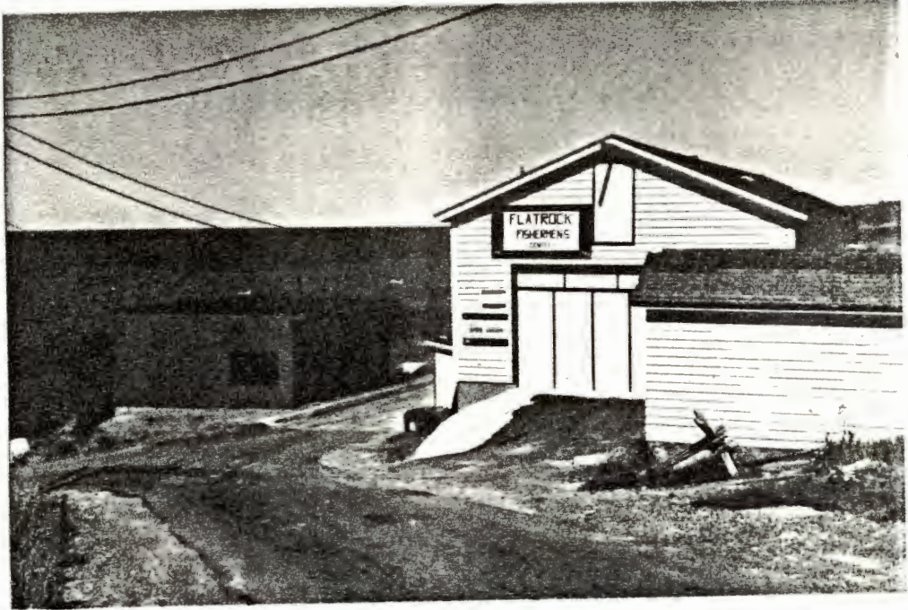
3. Fishermen's Center / Gear Storage Building
