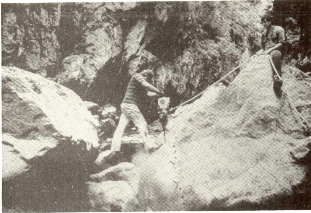
Figure 7. "Low level technology", such as stream clearance, is used to make inaccessible spawning and rearing habitat accessible to Atlantic salmon. Important increases in salmon populations can be achieved through such simple procedures.
