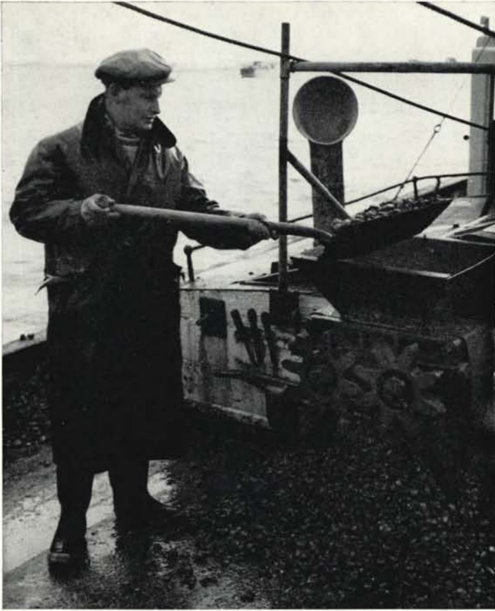
FIG. 44. An oyster fishing boat with a grinder installed for crushing old oyster shells and killing pests like mussels and slipper limpets. (Photo: P. J. Warren, after H. A. Cole, U. K. Ministry of Agriculture, Fisheries and Food.)
