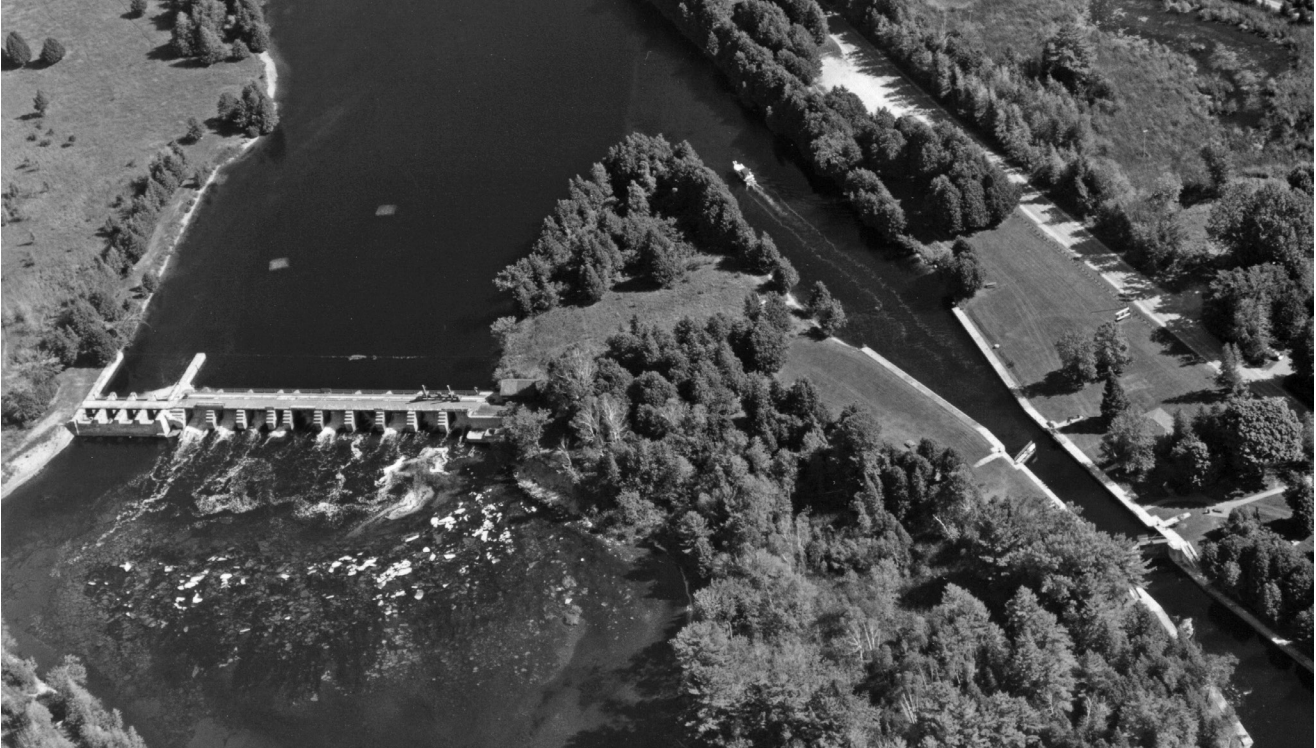
DOURO LOCK (LOCK 24) (2015)
