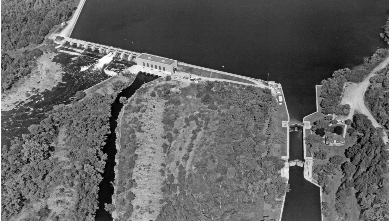
MEYERS LOCK (LOCK 9) (2015)
