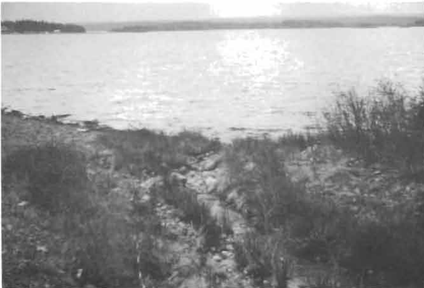
Figure 13. One of several drainage ditches carrying run-off from the Trans-Canada Highway.
