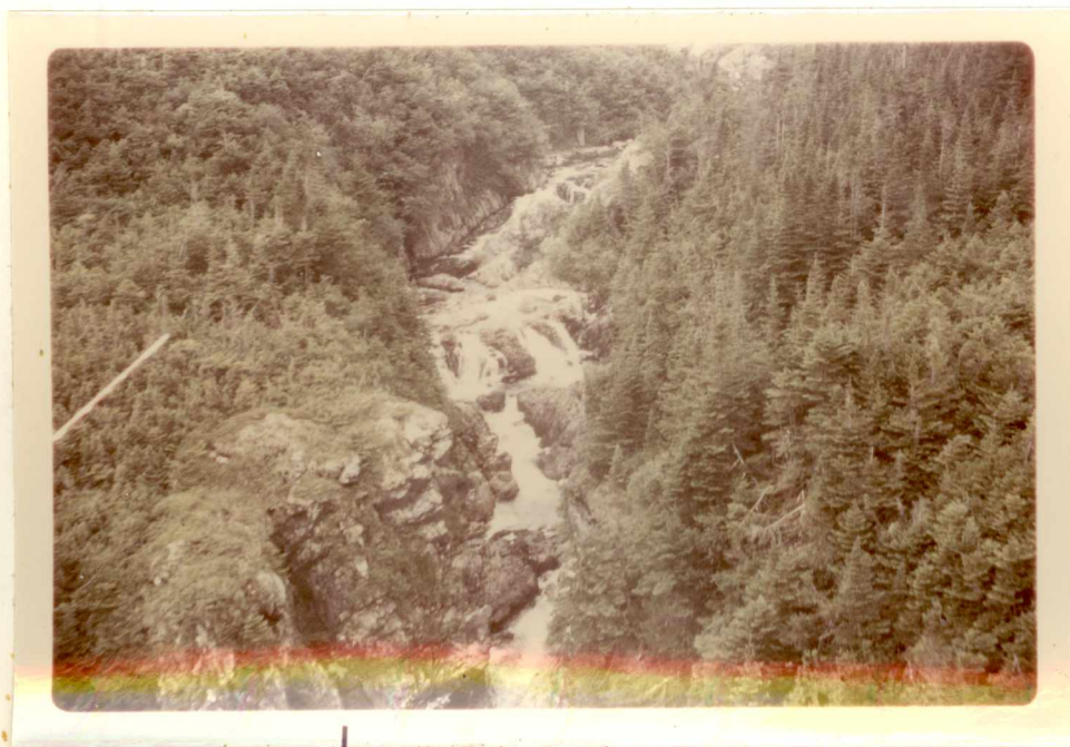
Fig. 52. Falls No. 2, Garnish River, complete except high water
