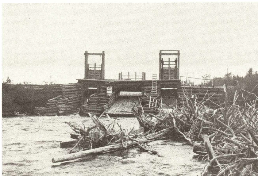
Typical logging dam on Exploit's River.
