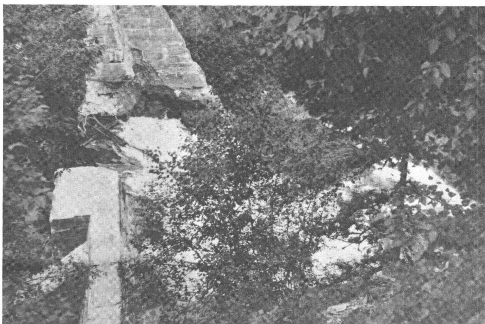
Side view of the concrete dam remnants.
