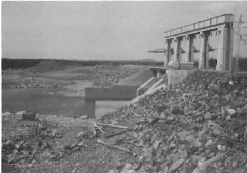
Fig. 3. Jacopie Control Structure (diverts water towards the forebay of the reservoir).
