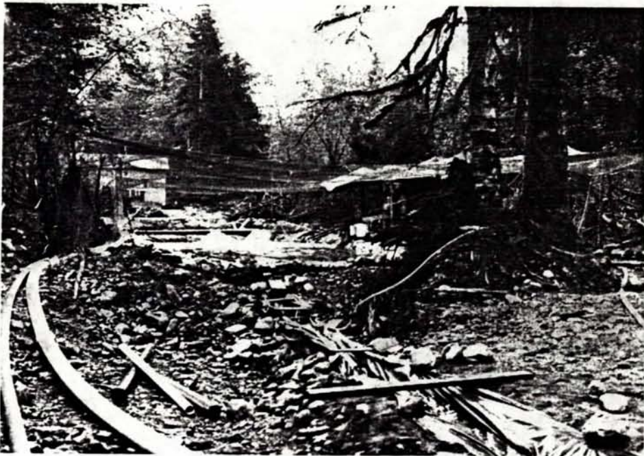
Fig. 11. Chinook rearing pond with overhead netting; plastic-lined outflow trough for carrying fish into Indian River is seen in foreground, 1980.
