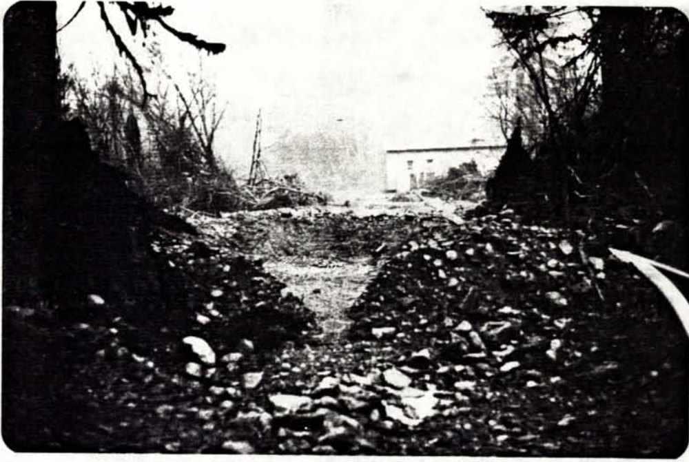
Fig. 10. Excavation of chinook rearing pond, Indian River pilot project, 1979 - 1980 (hatchery building is seen in background).
