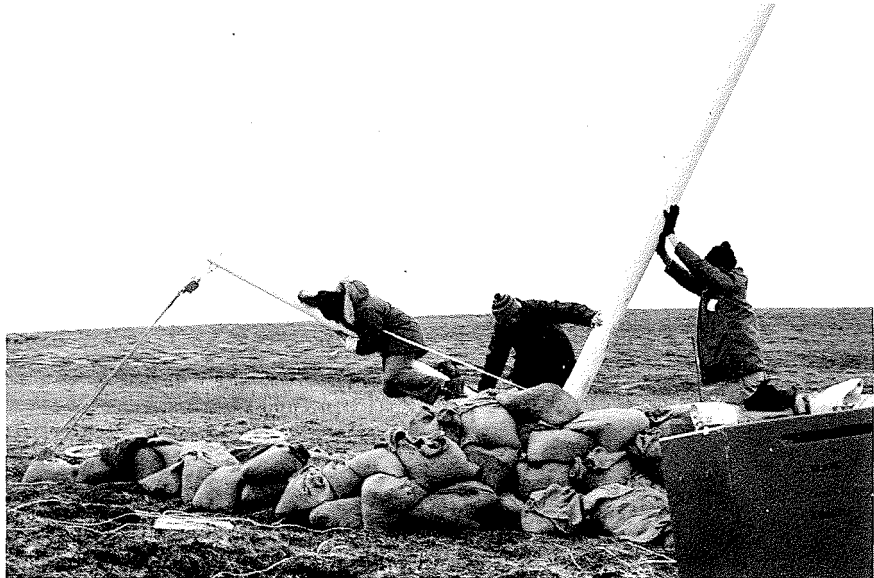
Hoisting a Minifix mast at Pullen Island, N.W.T.
