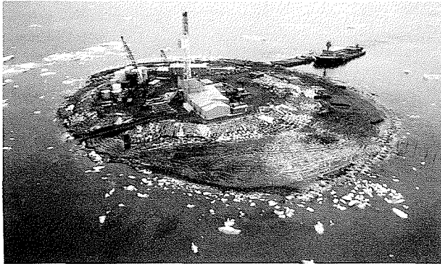
Beaufort Sea artificial island, needed for year-round drilling operation and production.
