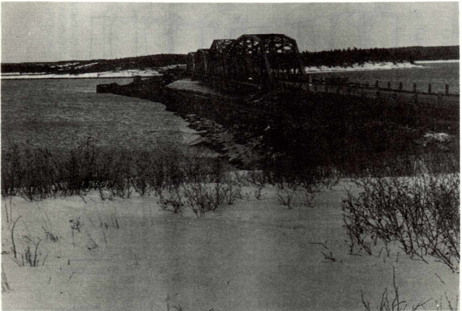
Fig. 24. View of Lennox Passage with dams under construction.
