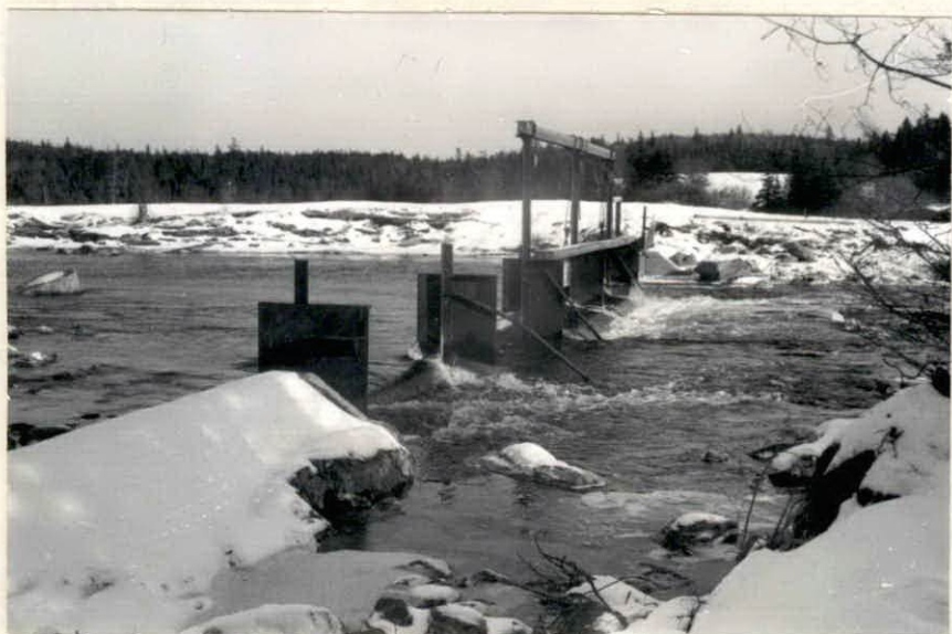
3 - Lower or Mill Dam
