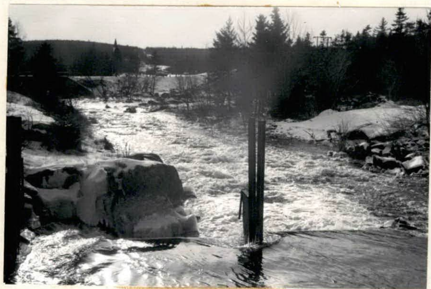
2 - Slasher Dam (1) looking downstream
