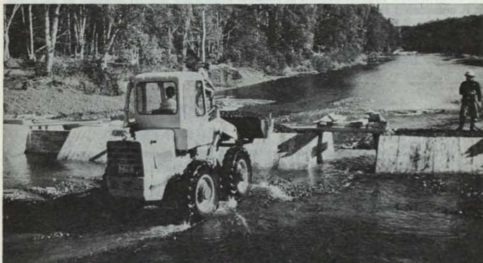
Weir construction, Indian River Spawning Channel, Newfoundland.
