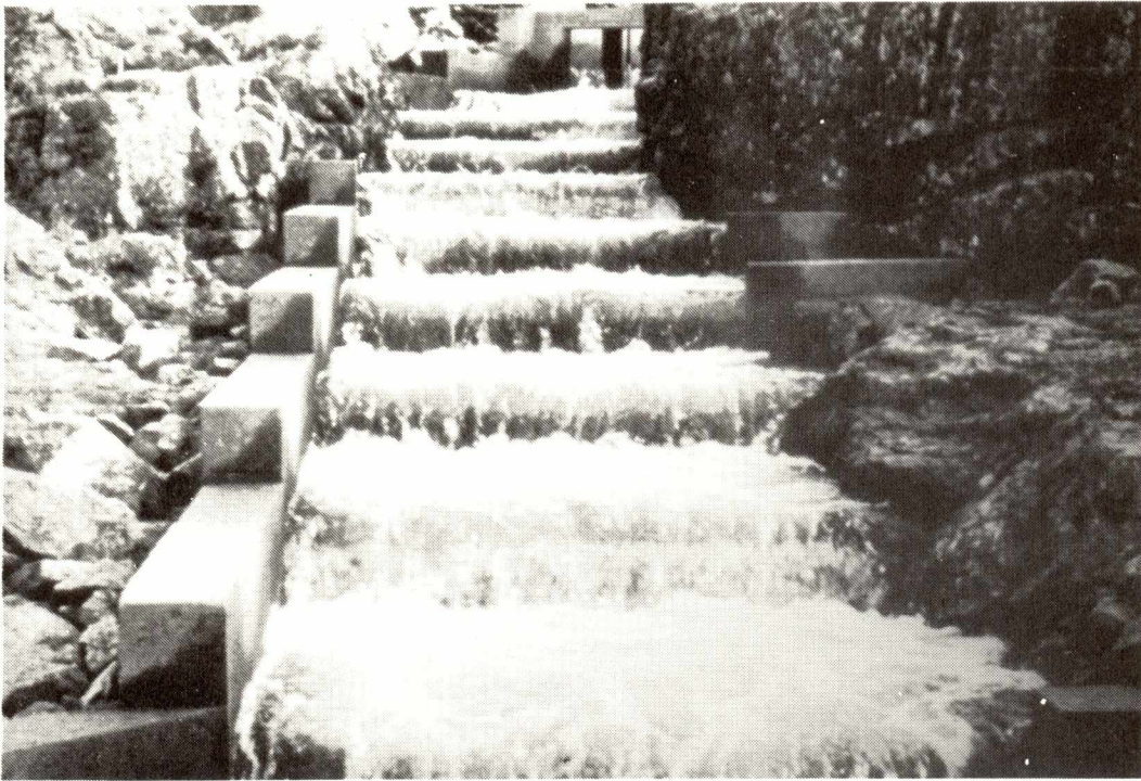
Figure 9. "Medium level technology" is required to allow salmon populations to expand into areas above more difficult obstructions. Results from the construction of this fishway (see Fig. 1) serve as a model for the future of many salmon enhancement schemes in Newfoundland.
