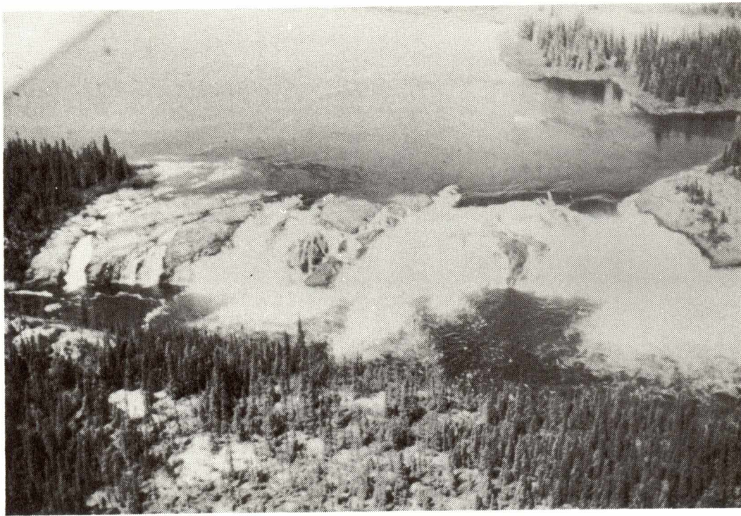
Figure 6. Numerous waterfalls in Newfoundland's wilderness areas are impassable to upstream migrating salmon. Many miles of fertile habitat would be available to expanded populations of salmon by installation of a fish ladder on the far left-hand side of this remote Labrador waterfall.
