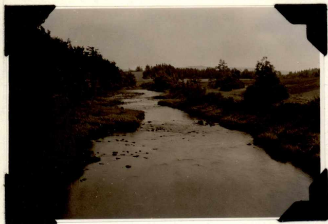
At Teed bridge.
