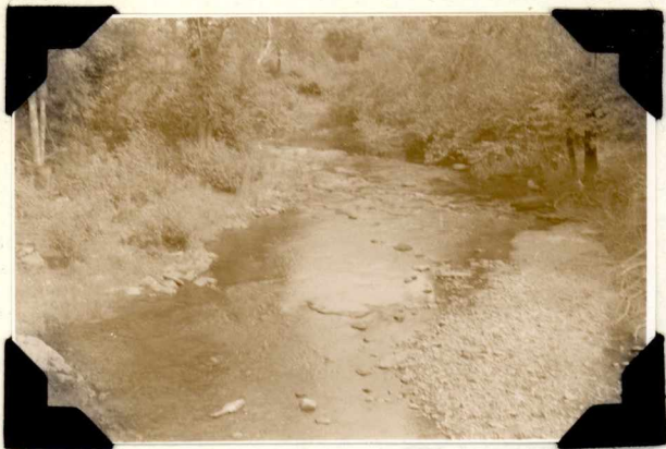
Near 2nd road bridge on East Branch.
