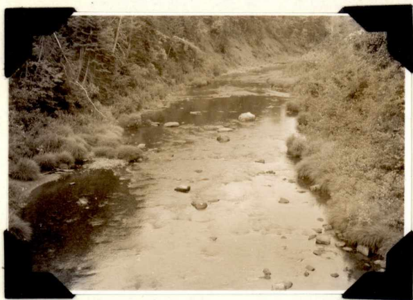
At Hunter bridge on West Branch.
