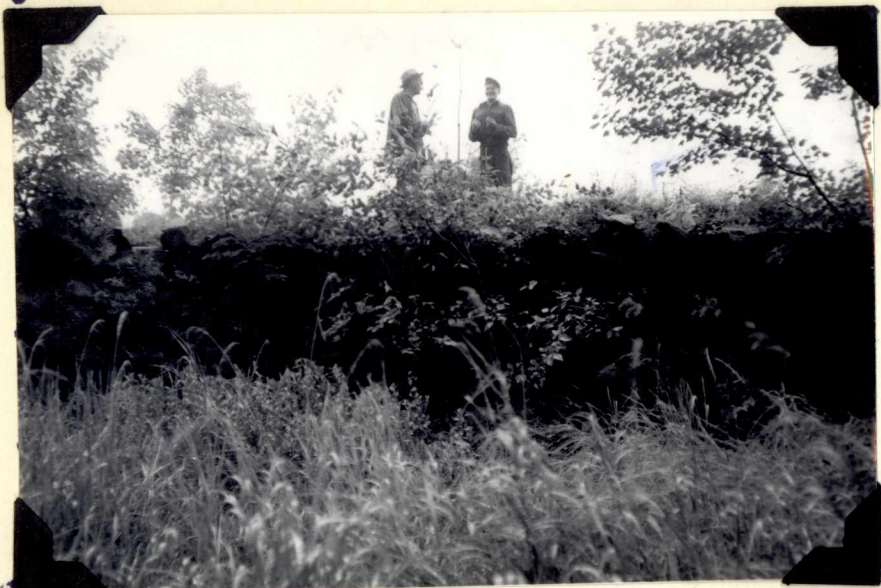
Above: Close up view taken from below showing type of construction.
