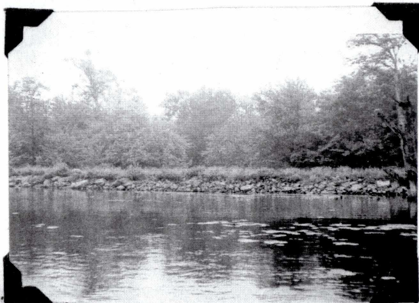
Approx. same section as above, taken from lake showing front of dam.
