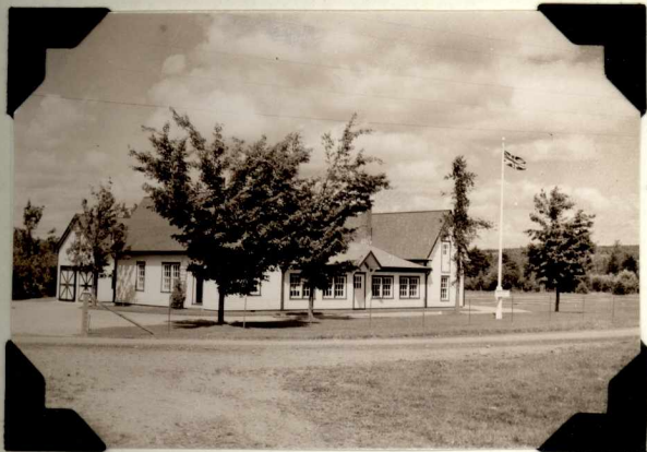
Hatchery buildings with entrance to premises to the left
