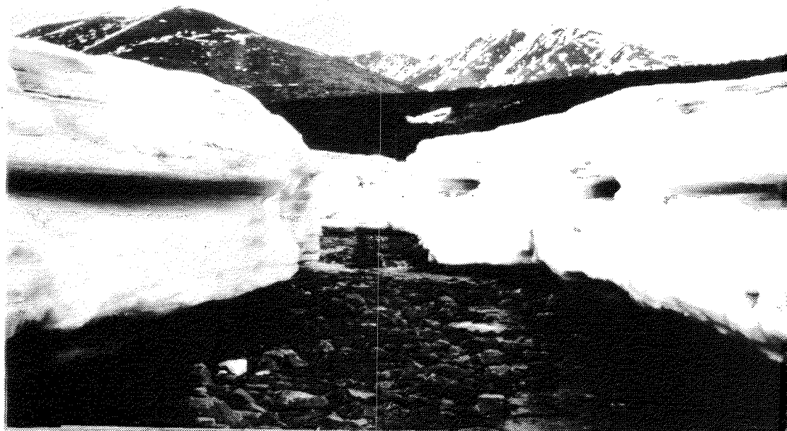
Figure 37. Formation of aufeis, and remnants of an aufeis deposit at a bridge crossing on the Dempster Highway, Yukon.
