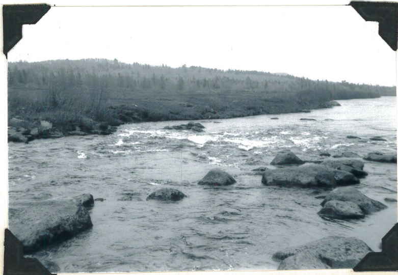
Fig. 12: Rapids below Crawford's Bridge. Blasting zone 2 looking downstream.
