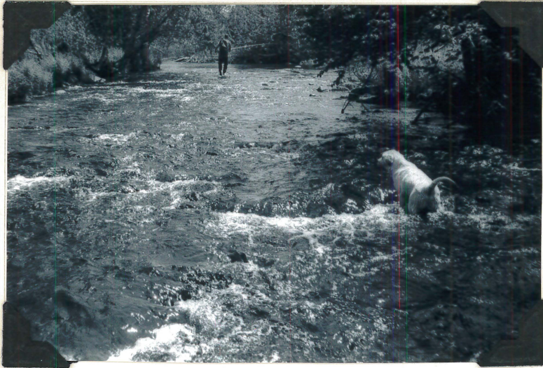
Fig. 27: Dam site #14 South Branch Musquodoboit R.
