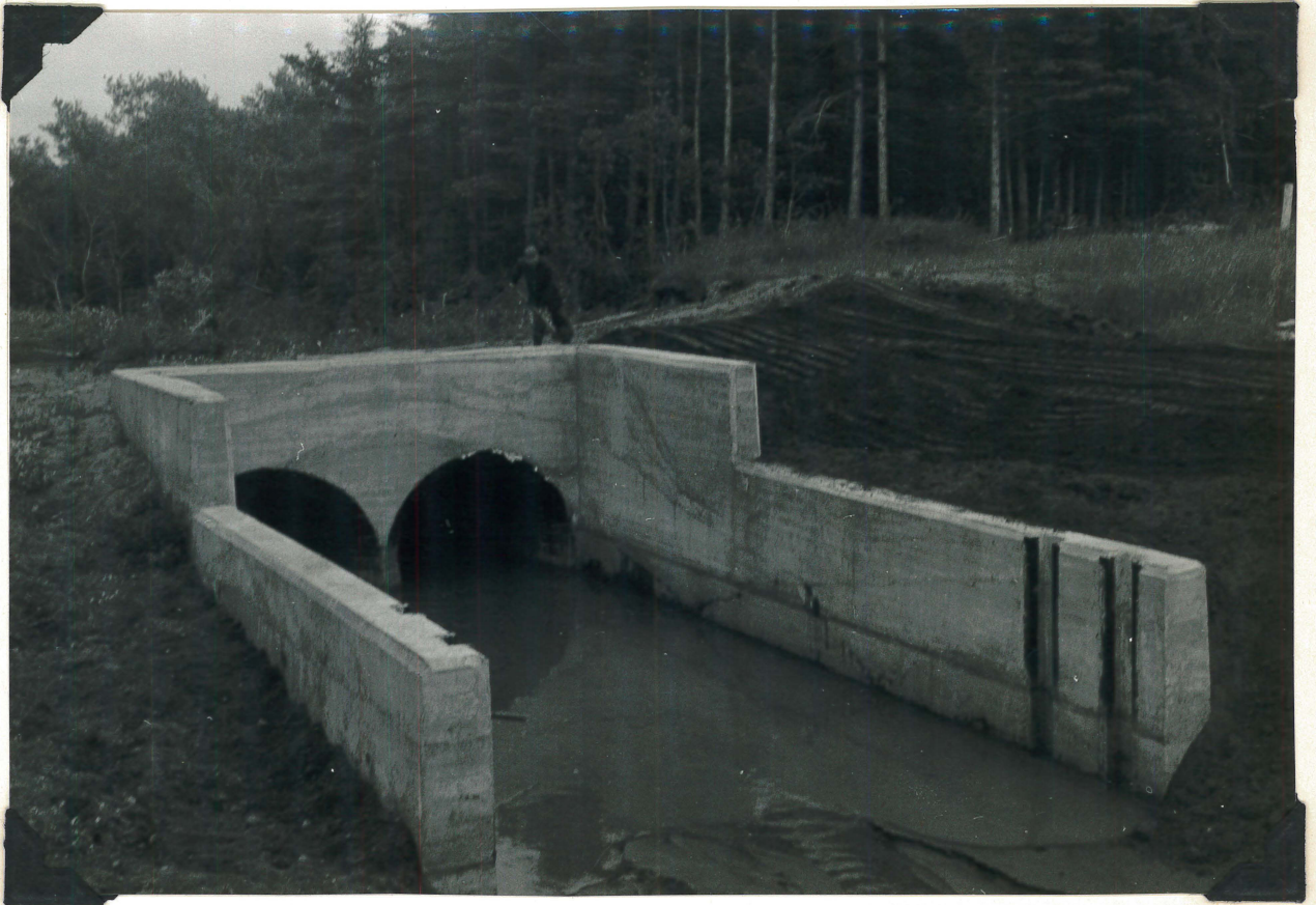
Fig. 35: Illustrating the type of dam and spillway to be used on the Musquodoboit water control program.
