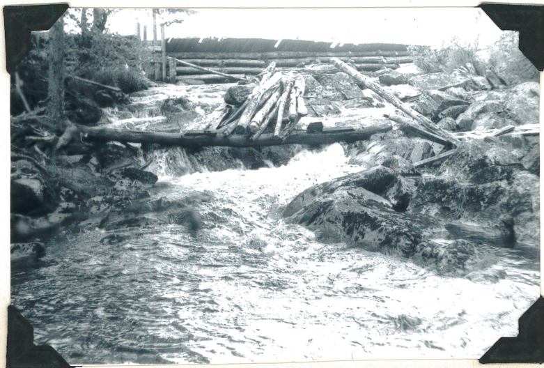
Fig. 16: Beaver Lake dam seen from downstream.
