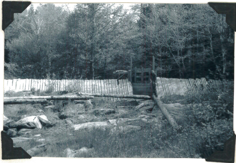
Fig. 15: The sluiceway gate in Beaver Lake dam.
