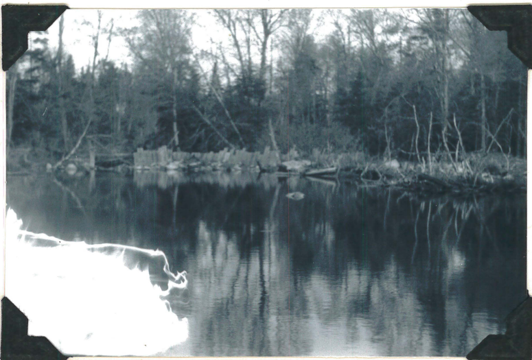
Fig. 29: Old logging dam on Ogilvy Brook above Beaver Lake (upper water- shed).
