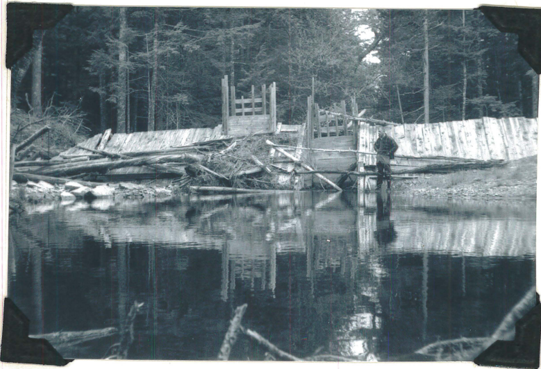
Fig. 31: Logging dam on Ogilvy Brook lower section above Beaver Lake. Dam is a total obstruction
