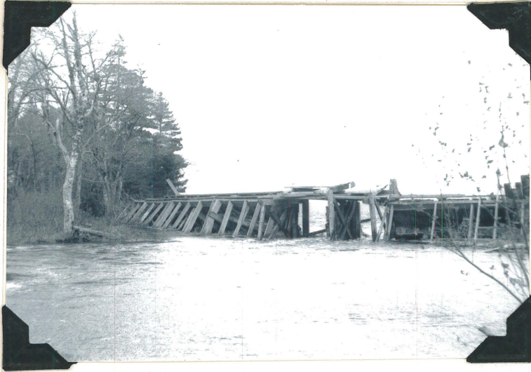
Fig. 7: Dollar Lake Dam viewed from downstream, gates are open.
