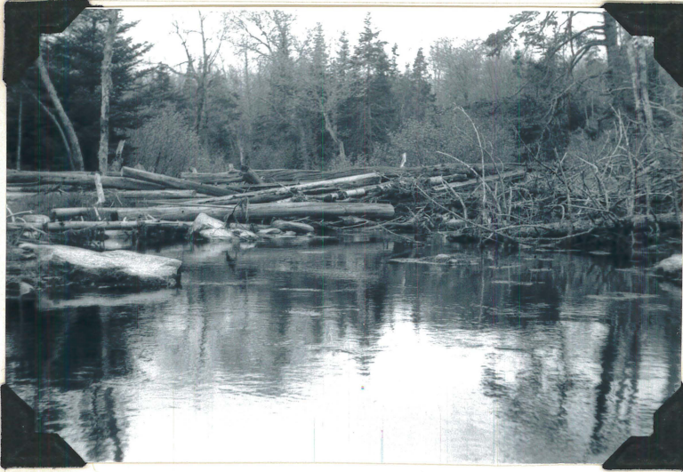
Fig. 30: Old logging dam on Ogilvy Brook middle section the dam is partly demolished
