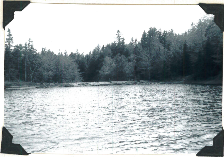
Fig. 14: Dam on Beaver Lake outlet. Dam site #3
