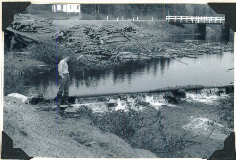
Fig. 33: Retention dam at Carter's Mill on Ogilvy Brook near the mouth.
