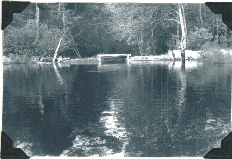
Fig. 25: The dam at lower Mill Lake outlet. Dam site #11.
