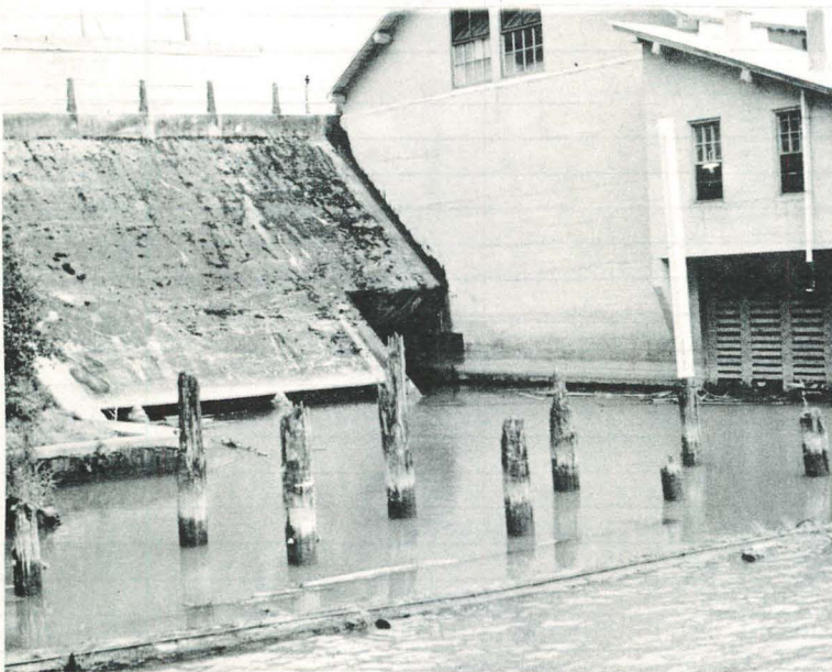
Sumas River looking upstream toward pump house.
