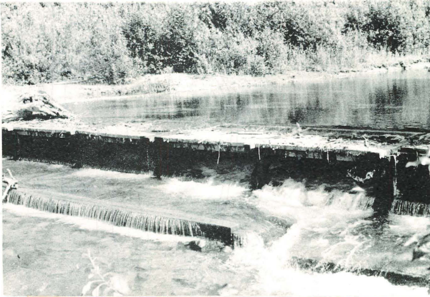
Wahleach Creek - fish diversion weir
