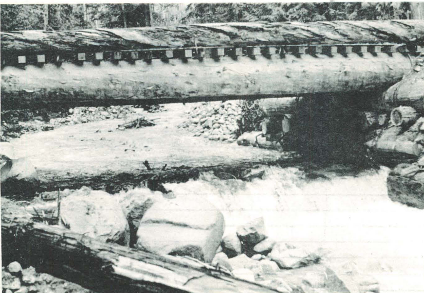
Paleface Creek looking upstream at logging bridge
