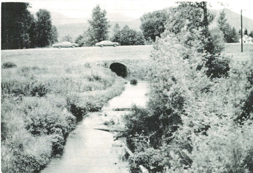
Luckakuck Creek - upstream towards freeway
