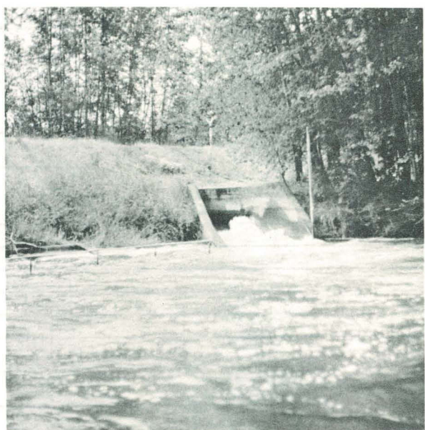
Downstream side of pump house on Chilliwack Creek.
