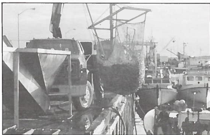
Herring being unloaded using the net bag system (Shippagan, New Brunswick) — A one step operation
