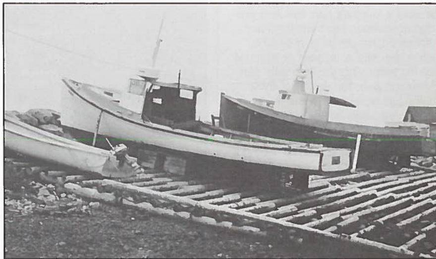
One type of ramp used to "dry dock" small vessels (up to 44ft.) in the Maritimes.
