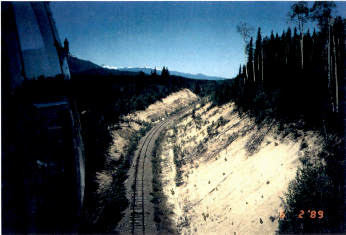
Figure 6.9 British Columbia Railway near Middle River showing typical construction cut and associated bank erosion issues. Photo courtesy of B. MacDonald.
