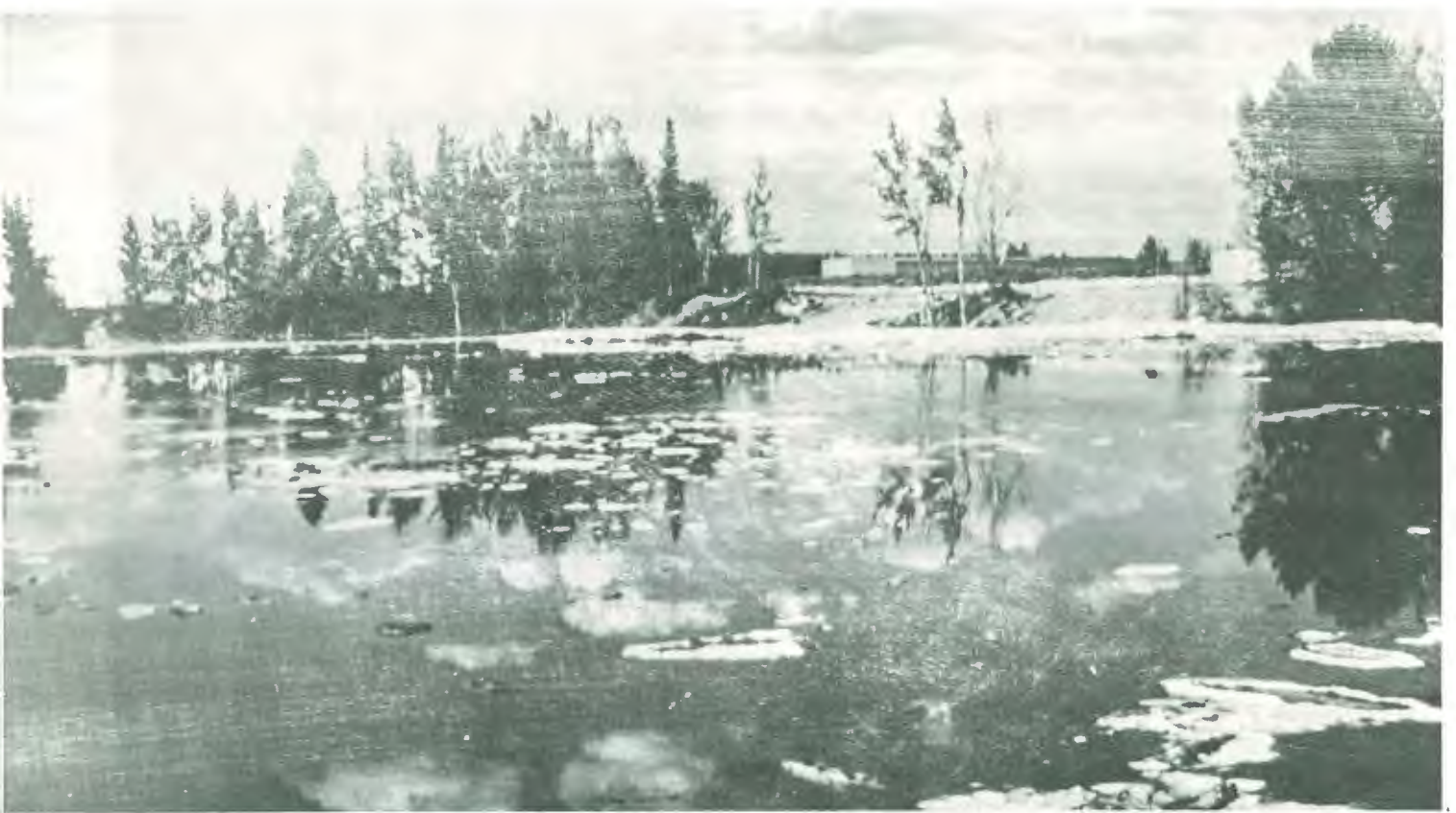
Biological-treatment pond for oil refinery effluent. Froth on water surface indicates aerator in action.
