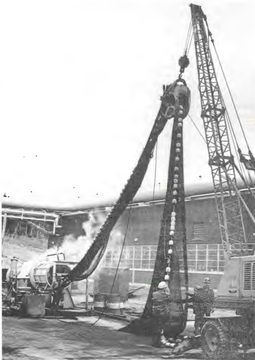
The steam laundry specially constructed to clean oil from seine nets, shown in action at Point Tupper, N.S.
