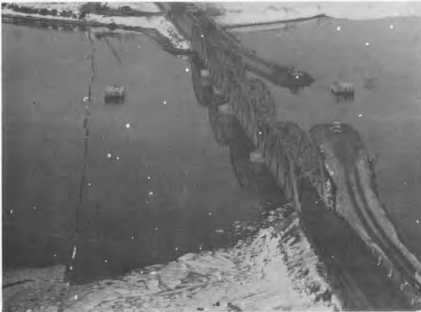
To contain the spread of oil at Lennox Passage, a boom of spruce boughs and chain link fencing was erected and a temporary dam constructed (seen at right of bridge).
