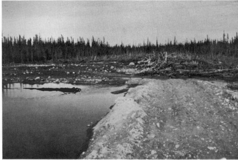
Figure 19. Tailings flow around the end of the east-west dyke, Pine Point, N.W.T., 1971.
