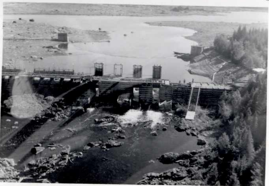
Figure 21: Main Dam Noel Paul Brook (Obst. 47)
