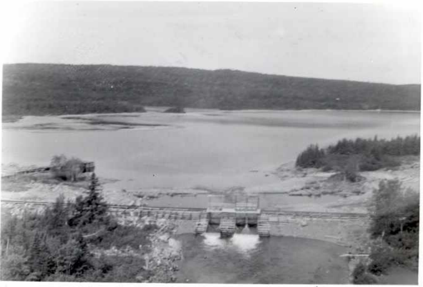
Figure 19: Main Dam Badger Brook (Obst. 38).
