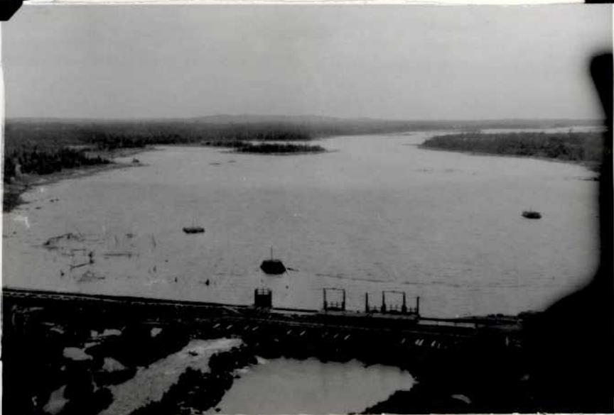
Figure 15: Main Dam on Sandy Brook (Obst. 11)
