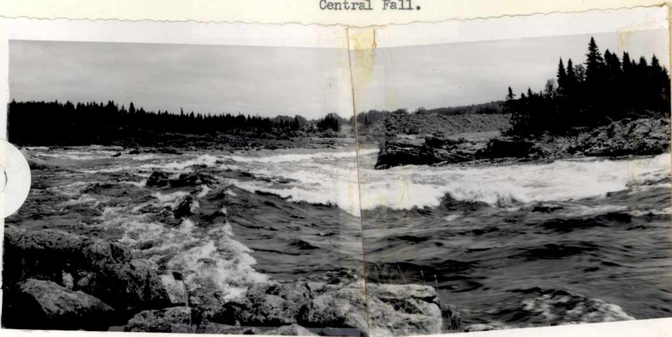
Figure 8b: Upper Grand Falls Obstruction - Central Fall.
