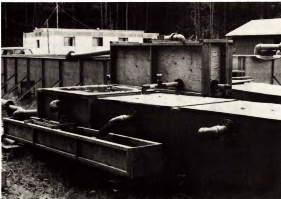
Fig. 12. Gravel incubation boxes with fry outflow trough in the foreground, Mathers Creek pilot hatchery, September 1984.
