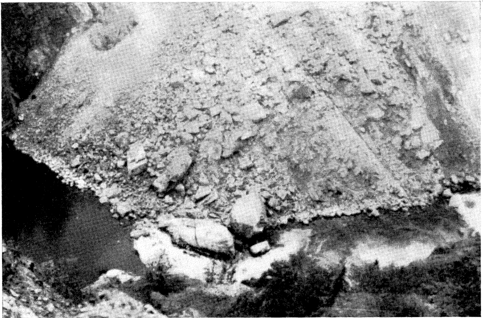
Figure 8. View of the lower part of the Slide, from the top of the cliff on the right bank, September 6, 1952. The upper rock was removed on August 27, leaving only two large rocks at the toe of the Slide.
