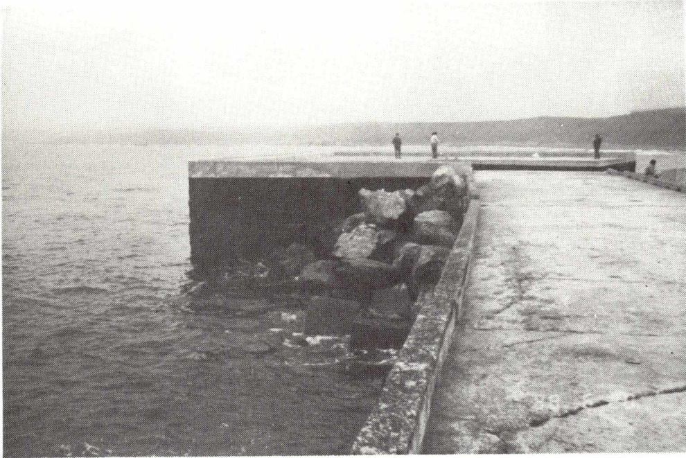
ST. BRIDES BREAKWATER REPAIRS
