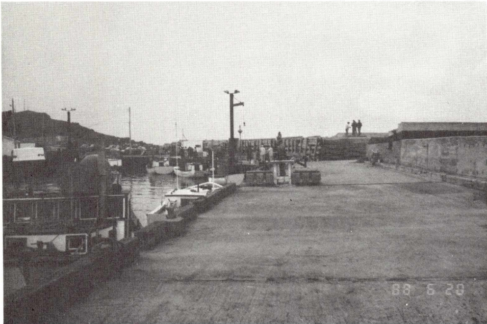
ST. BRIDES BREAKWATER REPAIRS
