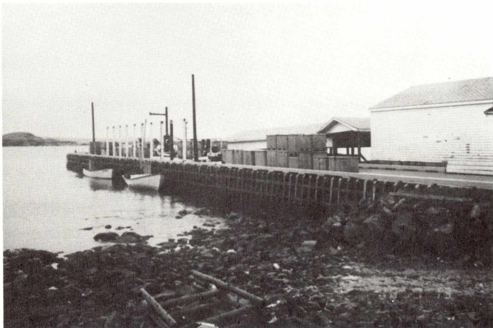
ST. LUNAIRE WHARF RECONSTRUCTION
