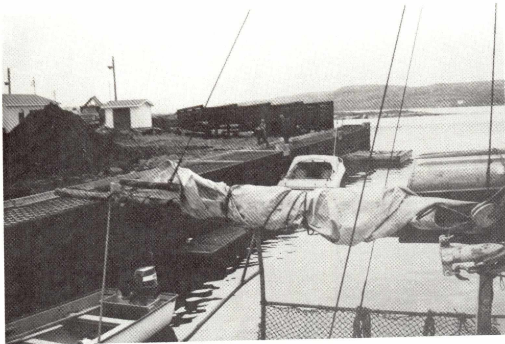
PUNCHBOWL MARGINAL WHARF CONSTRUCTION
