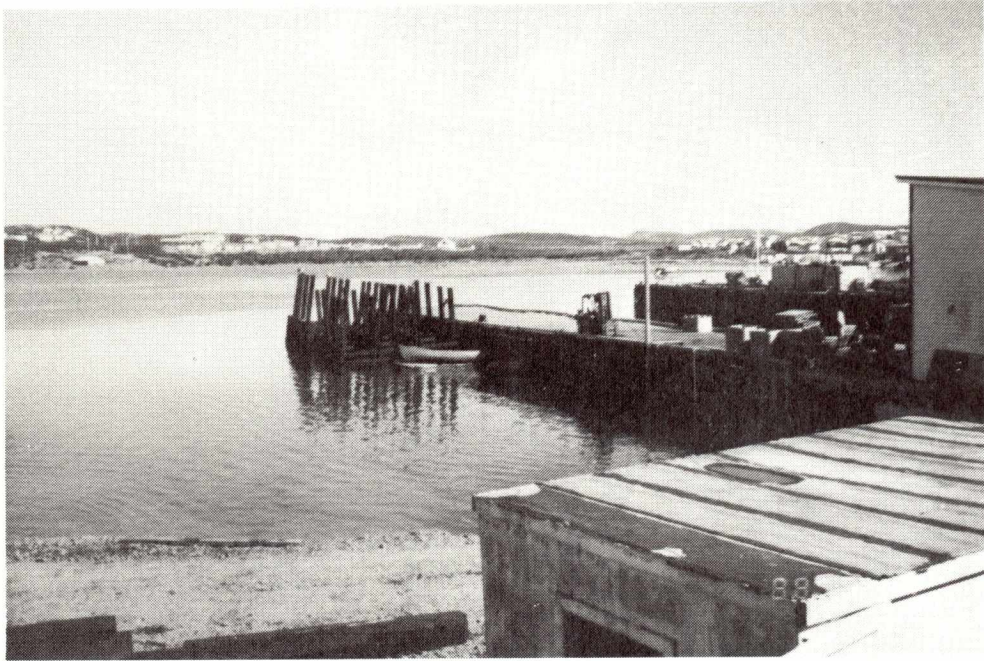
ARNOLD'S COVE WHARF CONSTRUCTION
