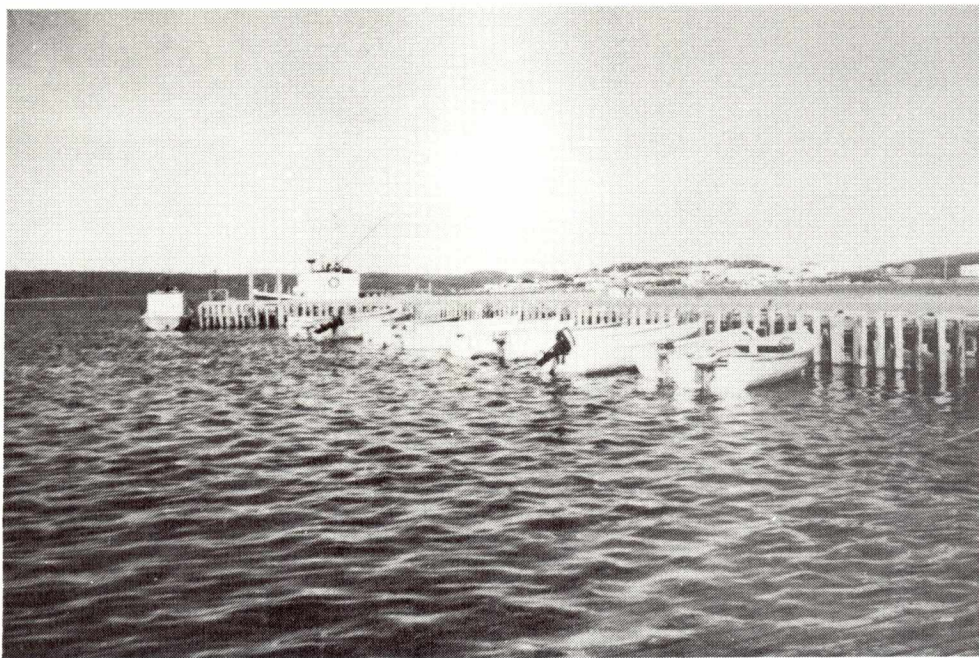
CENTREVILLE WHARF REPAIRS
