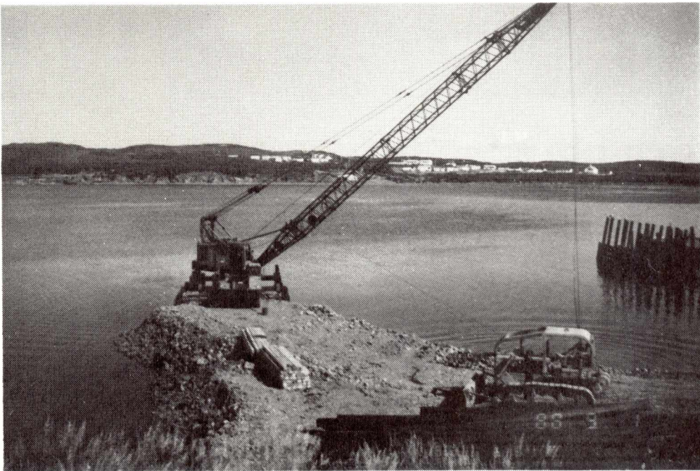
ARNOLD'S COVE WHARF CONSTRUCTION
