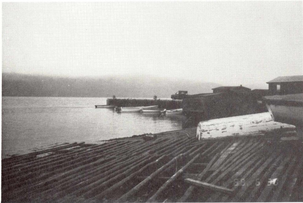
PRINCETON WHARF RECONSTRUCTION
