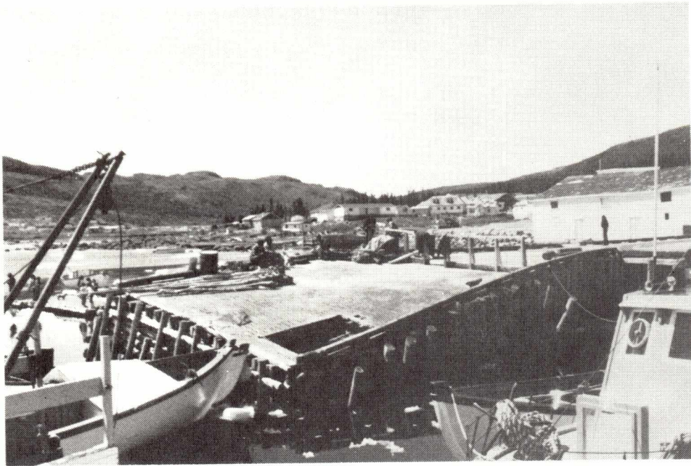
NAIN BEFORE WHARF RECONSTRUCTION
