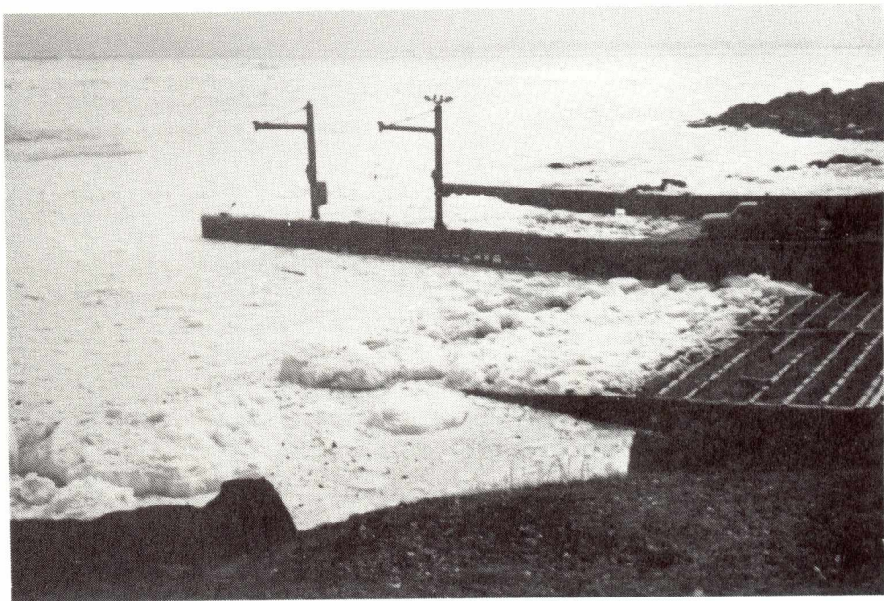
LOWER ISLAND COVE SLIPWAY REPAIR
