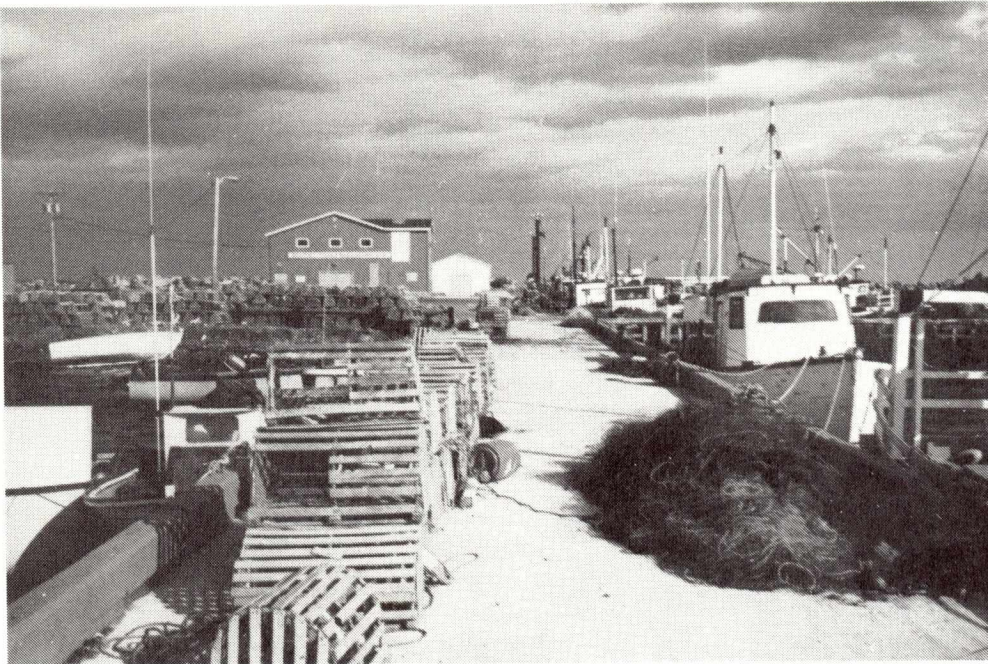
MUSGRAVE HARBOUR WHARF REPAIRS
