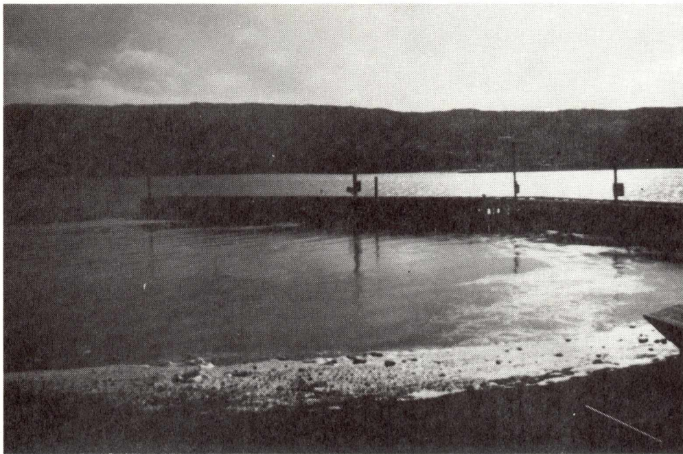
RIVERHEAD, S.M.B. WHARF REPAIRS
