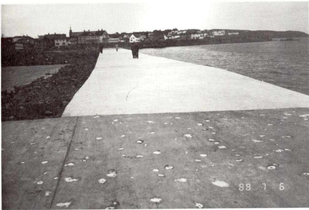
GRAND BANK BREAKWATER REPAIRS
