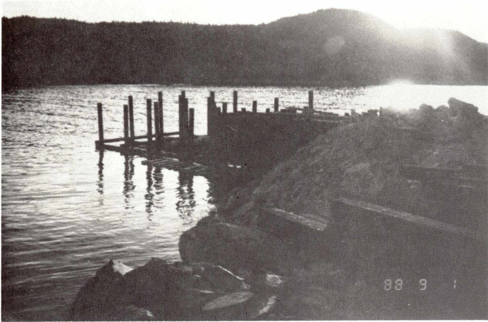
LA SCIE BREAKWATER CONSTRUCTION
