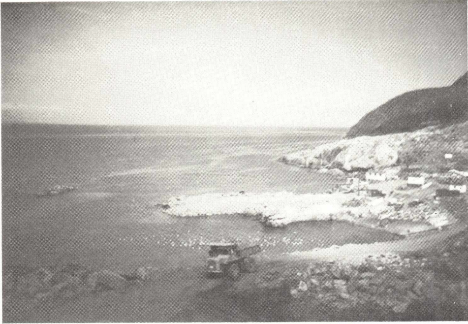
BAULINE BREAKWATER CONSTRUCTION
