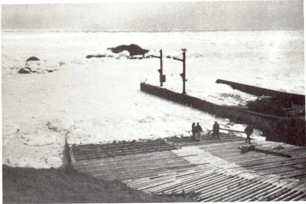
LOWER ISLAND COVE SLIPWAY REPAIR
