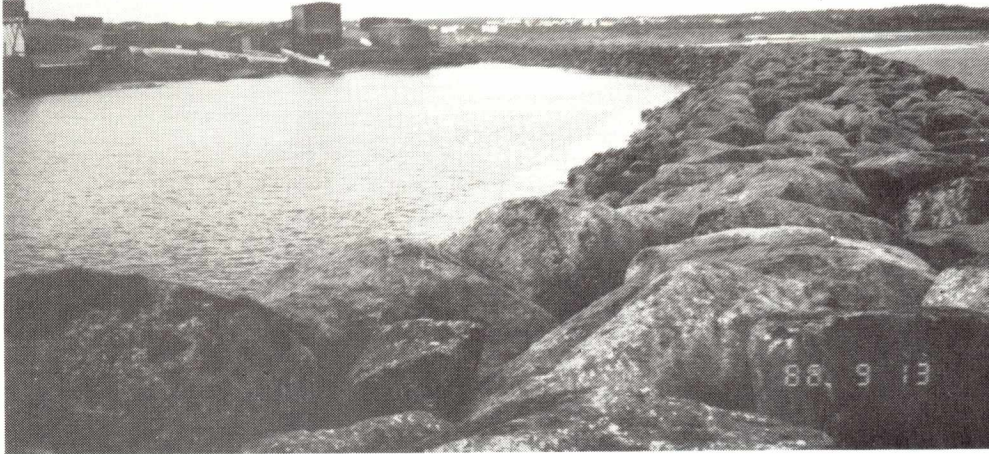
LUMSDEN SOUTH NEW BREAKWATER (LOOKING IN)
