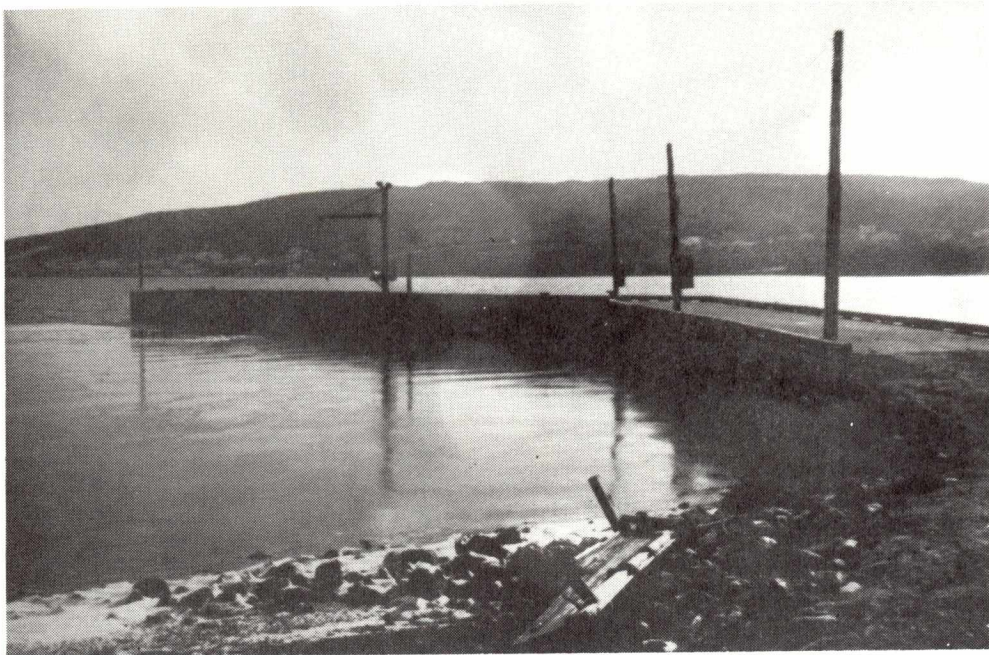
RIVERHEAD, S.M.B. WHARF REPAIRS
