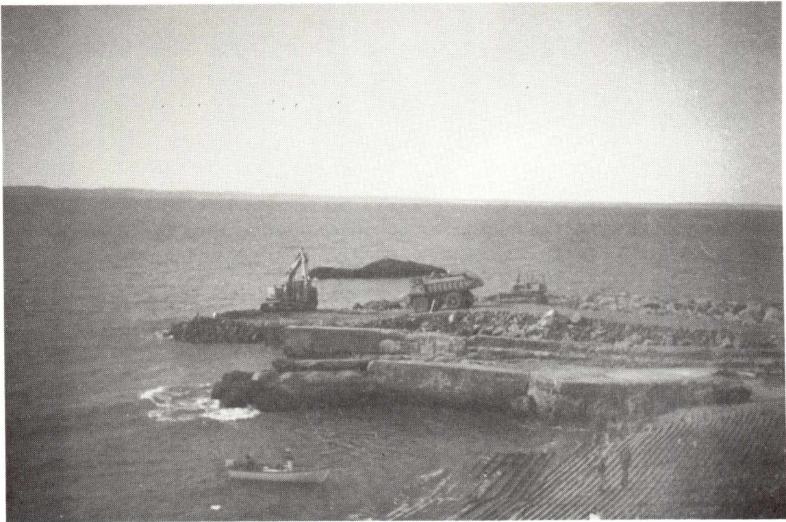
BAULINE BREAKWATER CONSTRUCTION
