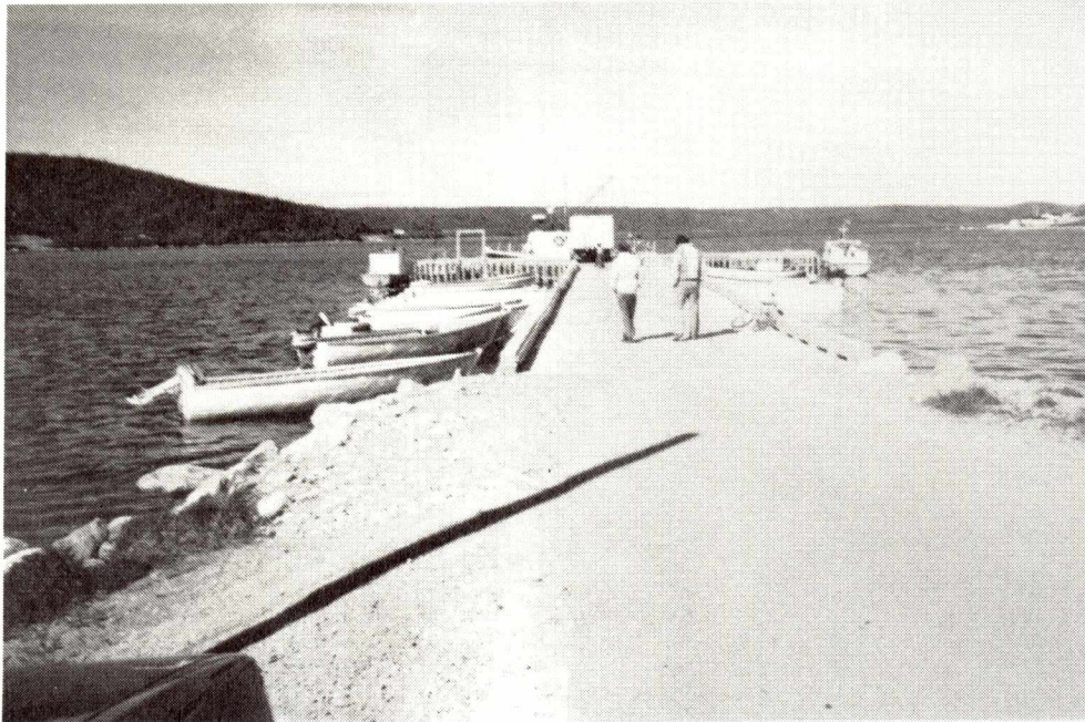
CENTREVILLE WHARF REPAIRS
