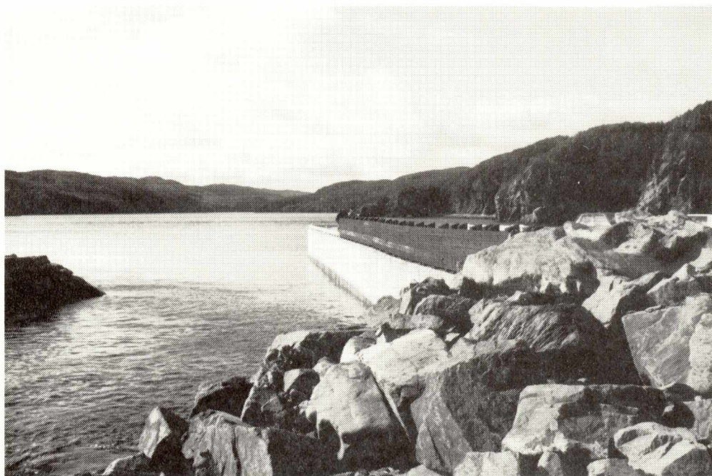
GOOSEBERRY COVE BREAKWATER CONSTRUCTION
