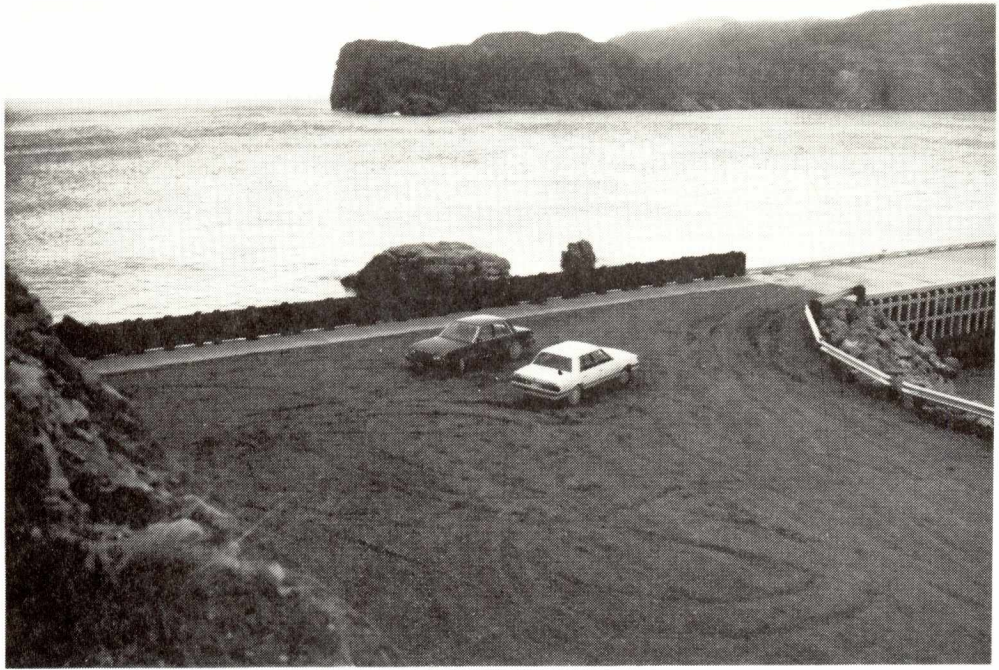
GOOSEBERRY COVE BREAKWATER CONSTRUCTION
