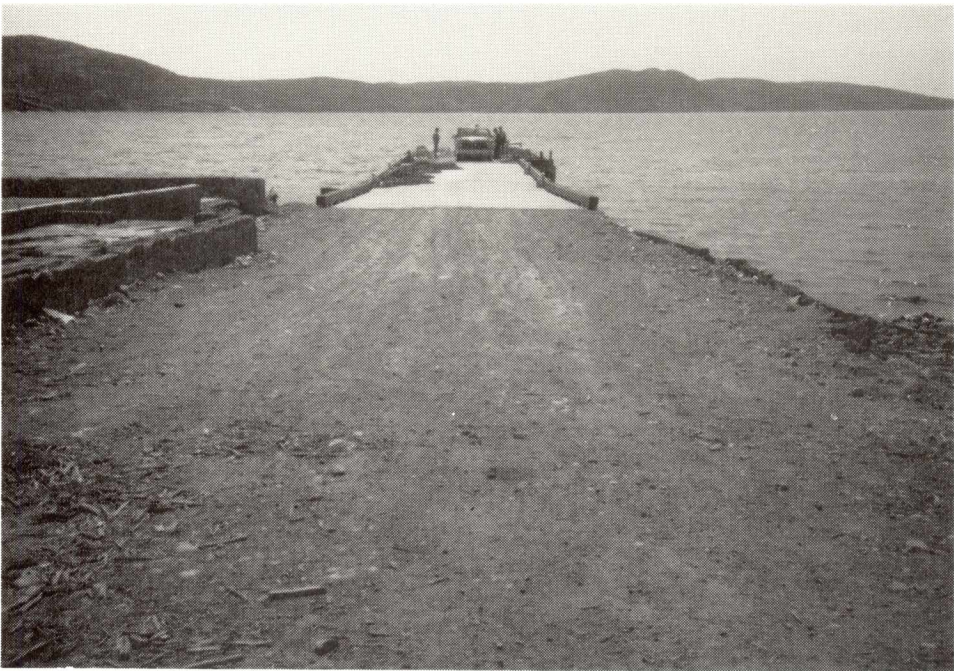
BONAVISTA (MOCKBEGGER) WHARF REPAIRS
