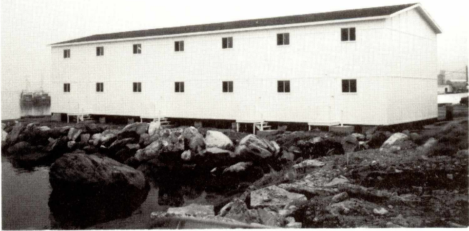
OLD PERLICAN GEAR SHED UNDER CONSTRUCTION (CANADA WORKS)
