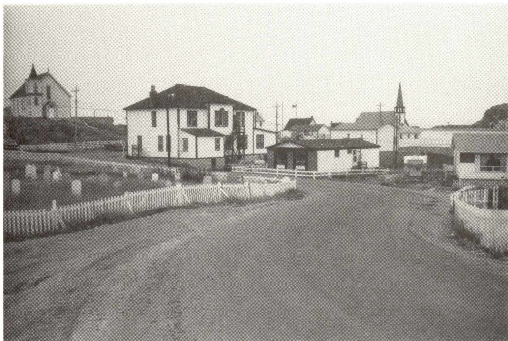
FOGO WHARF APPROACH PAVING
