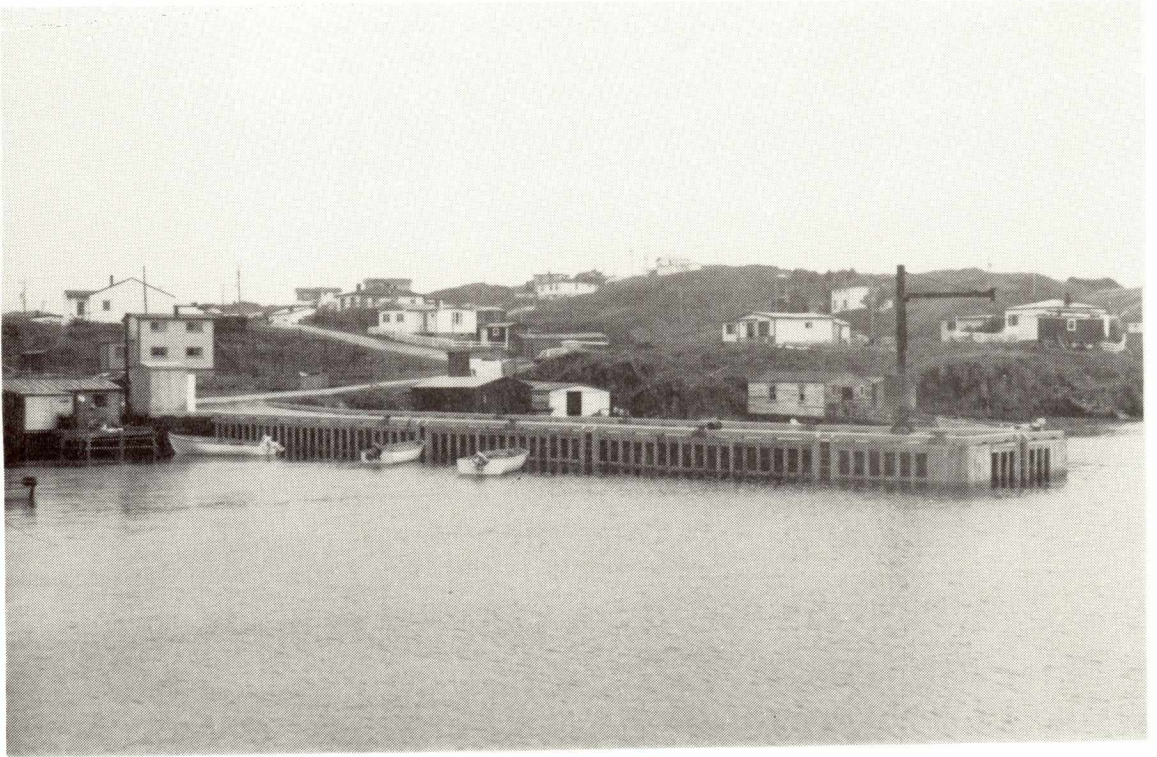
CHAMPNEYS WEST WHARF CONSTRUCTION (CANADA WORKS)
