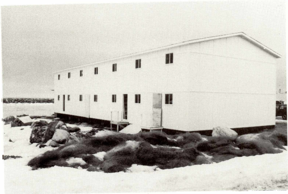
OLD PERLICAN GEAR SHED UNDER CONSTRUCTION (CANADA WORKS)
