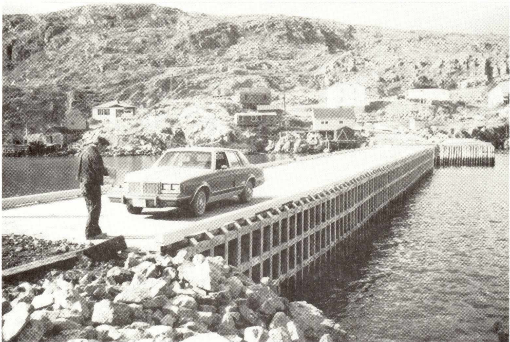
NIPPERS HARBOUR (NOBLE'S COVE) BREAKWATER RECONSTRUCTION
