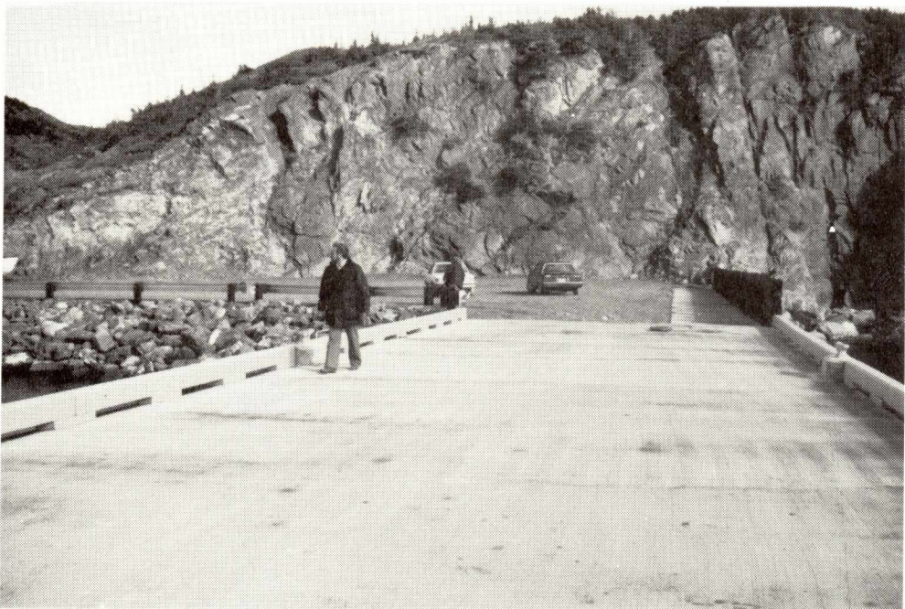
GOOSEBERRY COVE BREAKWATER CONSTRUCTION
