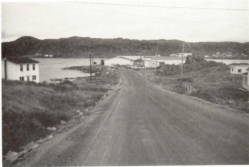
FOGO WHARF APPROACH PAVING
