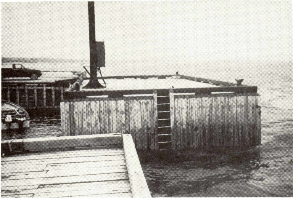
CAPE FREELS NORTH WHARF REPAIRS
