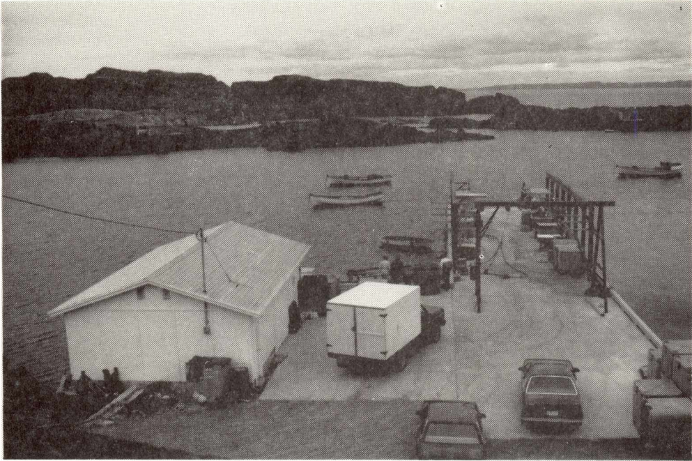
TICKLE COVE WHARF RECONSTRUCTION (CANADA WORKS)
