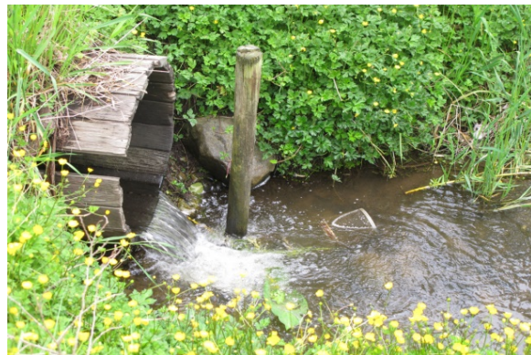
Figure 9. The single culvert draining Agassiz Slough to the Fraser River (Left, 2012) and a perched (hung) culvert draining an unoccupied tributary into potential Critical Habitat in Fishtrap Creek (Right, 2010).
